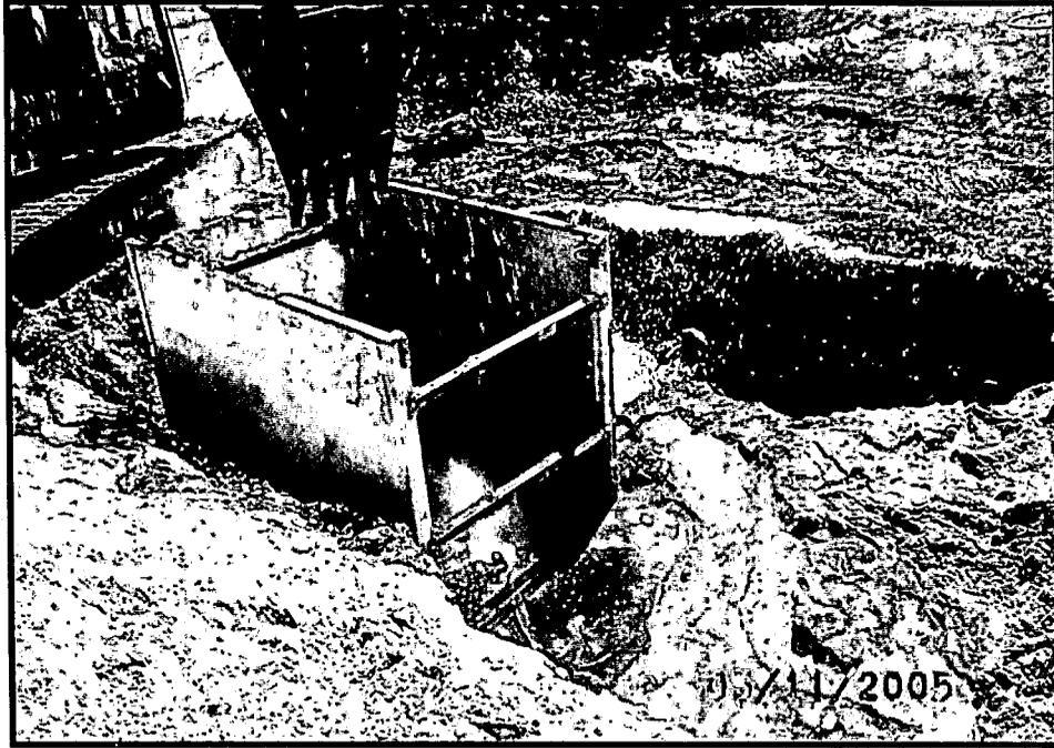
Excavation Area B – Excavation to 13 ft. bgs using trench boxes
