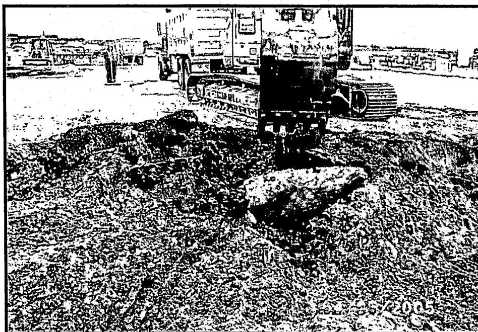
Excavation Area A - Tar layer 2.0 ft. bgs near asphalt road
