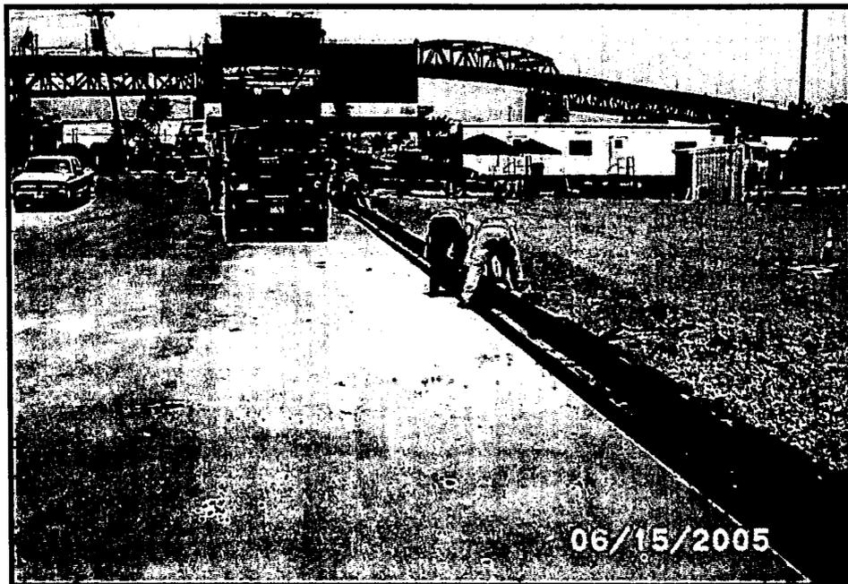
Crushed Stone Cap Area - Asphalt curbing on west side of cap
