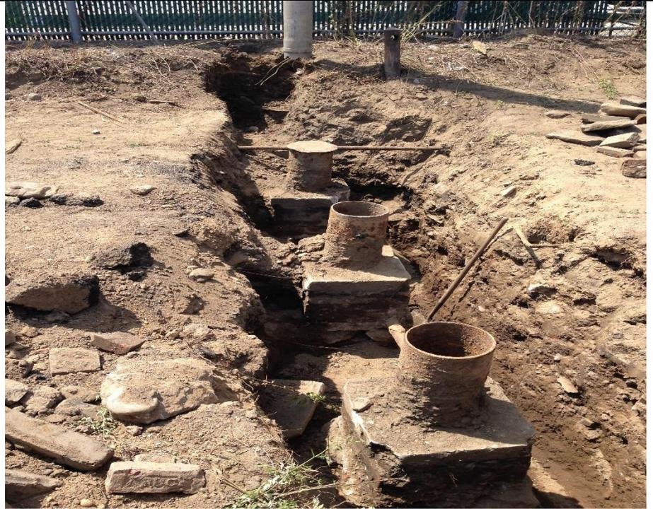
Photo 6 – Top westernmost valve port and fill or vent pipe on southern side of UST-1 area near site boundary fence and Vandervoort Avenue. Tank is accessible through small pipe visible in photo. Top of concrete vault approximately 4 feet below the top of the valve port.
