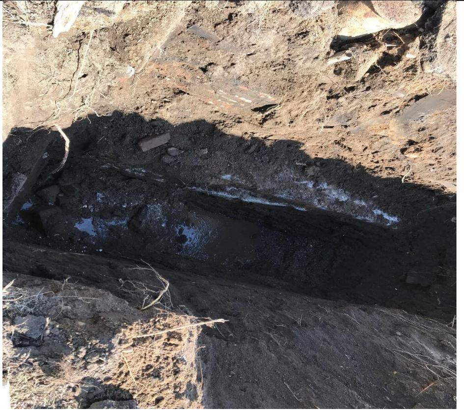
Photo 8 – Sheen shown on water in excavation south of UST-1 area.
