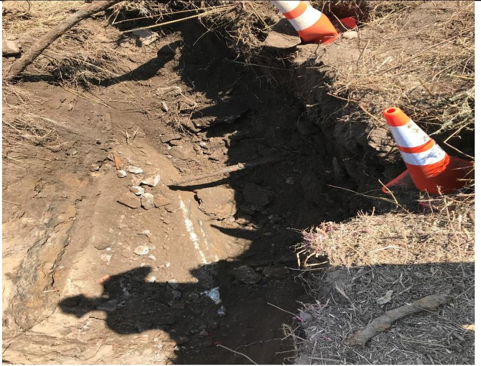
Photo 12 – Top of westernmost UST in UST-2 area near perimeter fence. Top of UST approximately 6 feet below grade.
