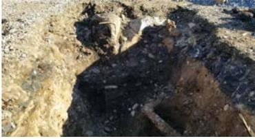
Photograph 2: Completed test pit, pipe and wall base.<br>
