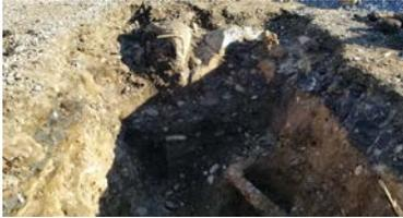
Photograph 2: Completed test pit, pipe and wall base.
