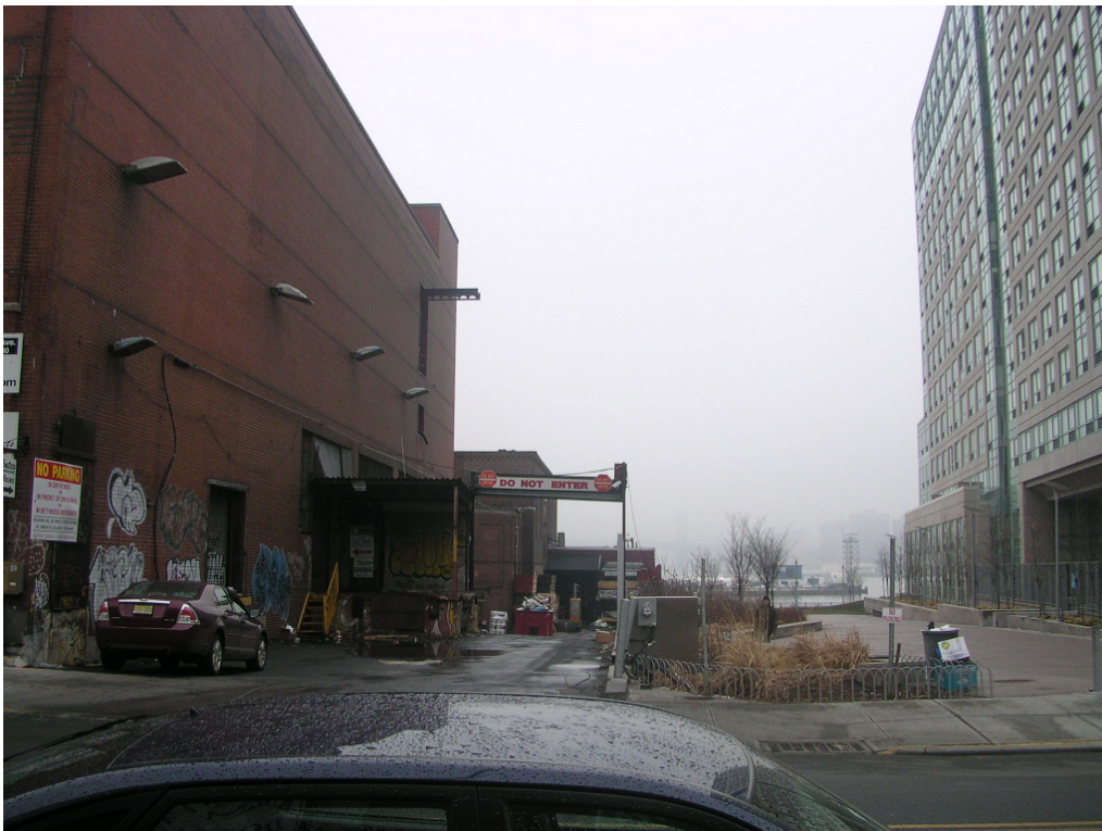
Photograph taken on April 2, 2007 from Kent Avenue of the northern side of the site looking west.
