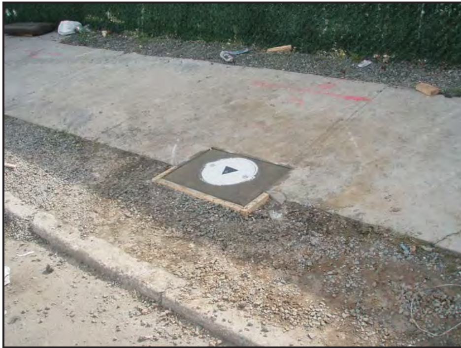
Photo 21: Completed well cover and concrete restoration.
