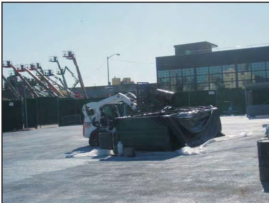
Photo 6: Rolloff for soil and concrete/asphalt.
