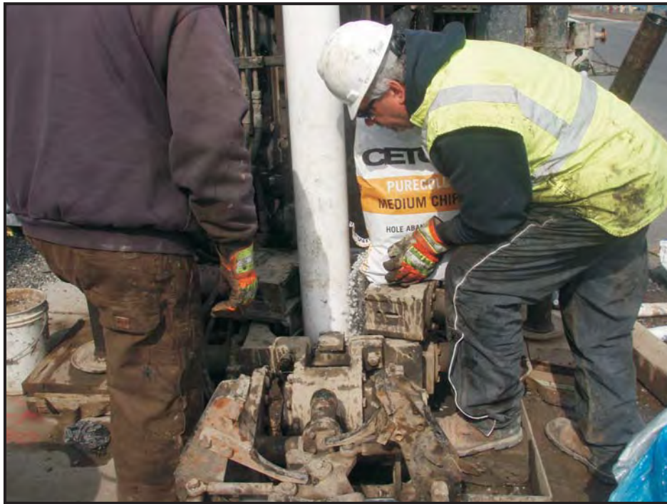
Photo 13: Bentonite chips poured into boring.
