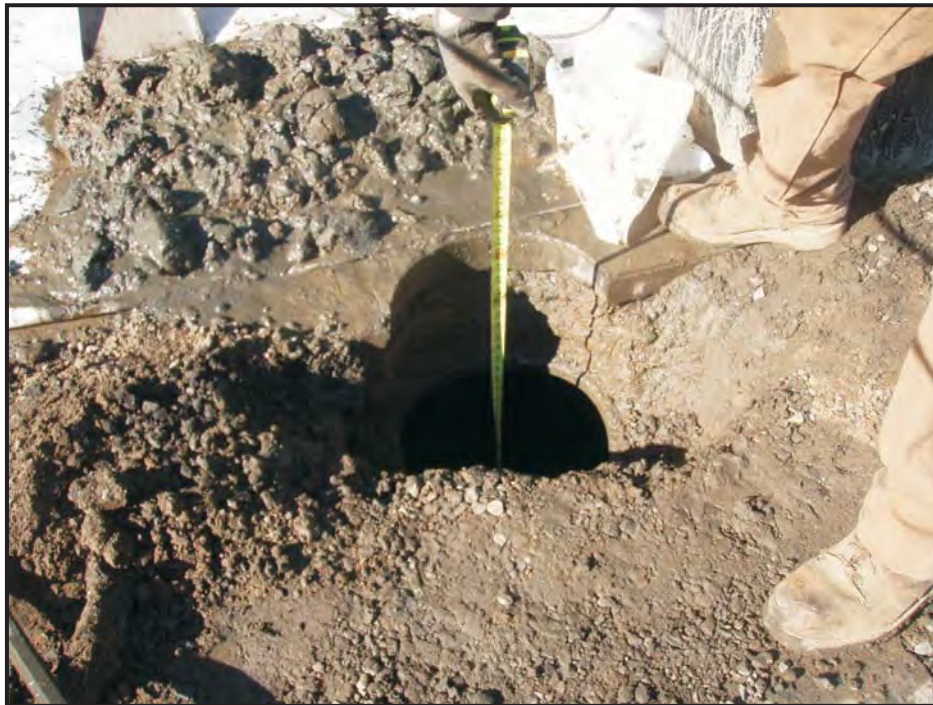
Photo 17: Cored hole through 24" gas line.
