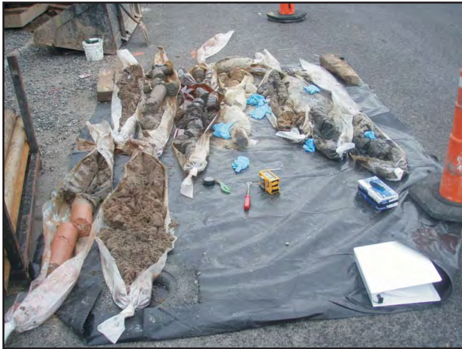
Photo 9: Continuous sampling during soil boring.
