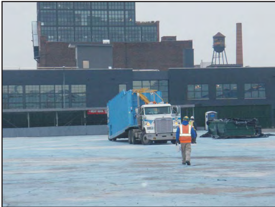
Photo 5: Delivery of water storage tank.
