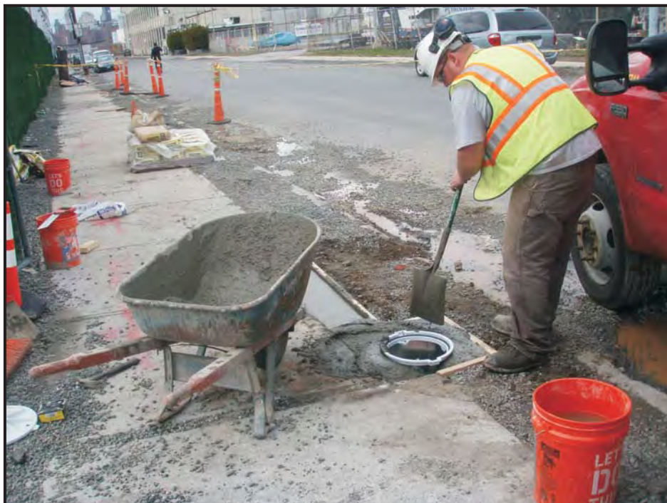
Photo 20: Placing cement around well cover and sidewalk restoration.
