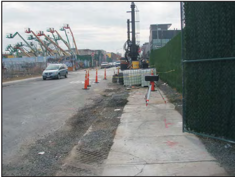
Photo 15: CAMP setup and traffic safety barriers.
