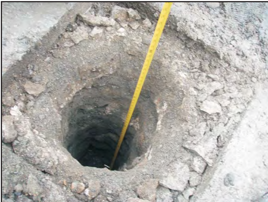
Photo 2: Precleared hole to 5 foot.
