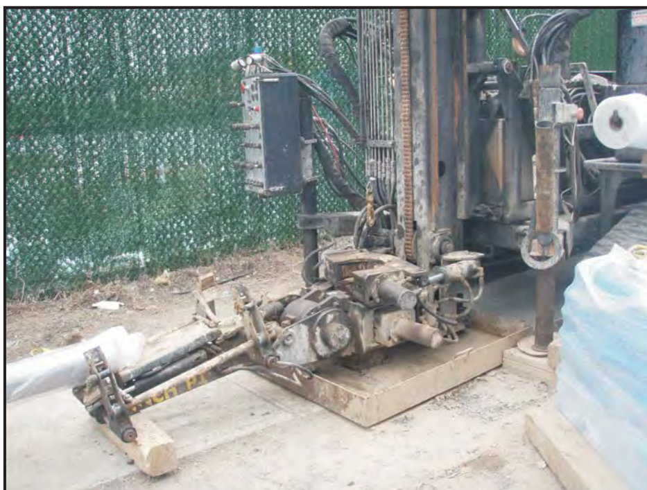
Photo 8: Sonic Drill Rig setup and collection pan.
