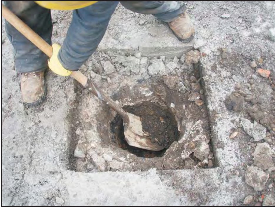
Photo 1: Preclearing well location to 5 feet.
