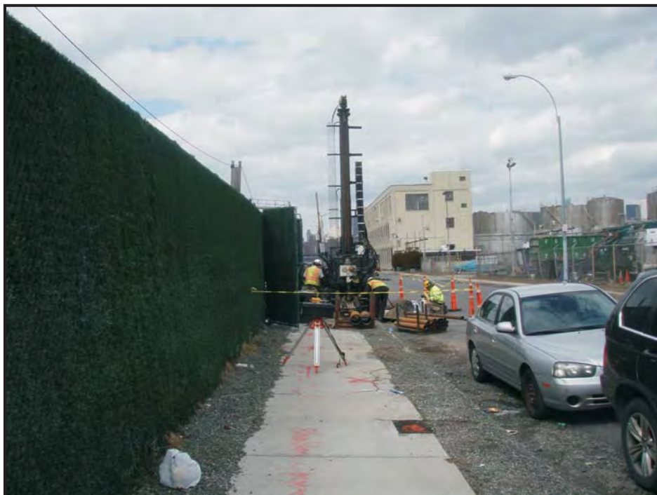
Photo 14: CAMP setup during drilling.
