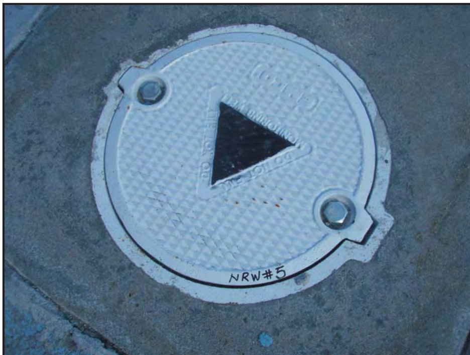
Photo 22: Completed well cover.
