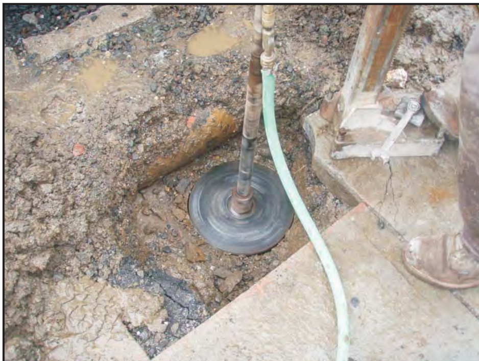
Photo 16: Coring 24" inactive gas line along N. 12 th Street.
