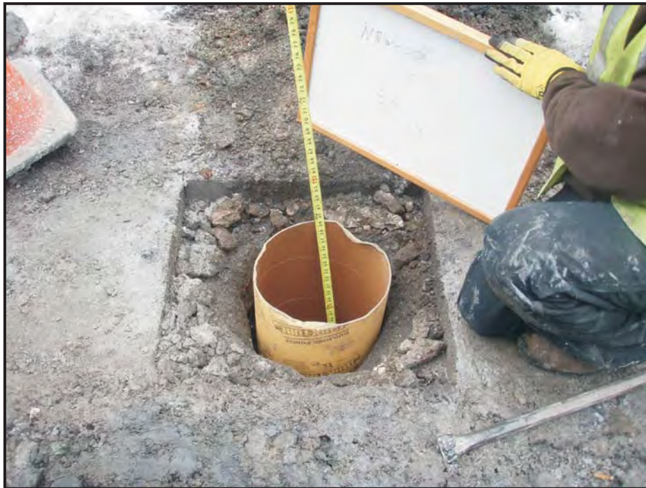
Photo 3: Precleared hole to 5 foot.
