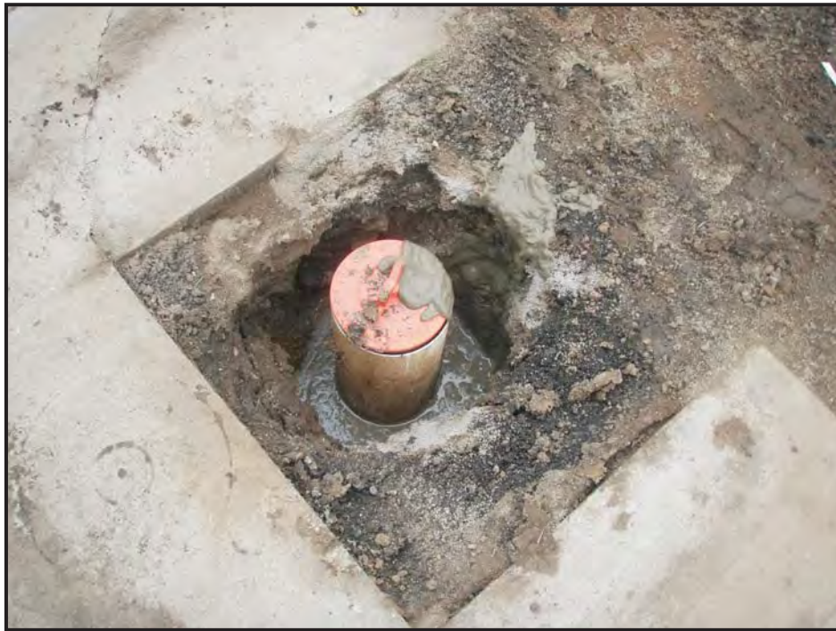
Photo 19: Well plug installed after well installation and grouted.
