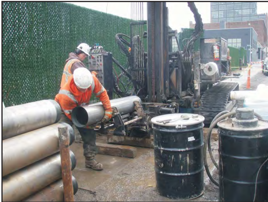
Photo 7: 10" drill casing for drilling bore hole.
