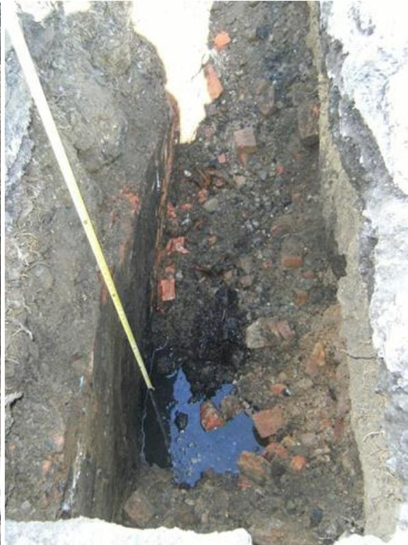
The December 2014 field investigation described in Section 1.2.4 provided additional information for refinement in the 100% design. Specifically, the depth of the perimeter wall was measured by drilling through the wall. This information was used to decide to demolish the perimeter wall during installation of SOE.
