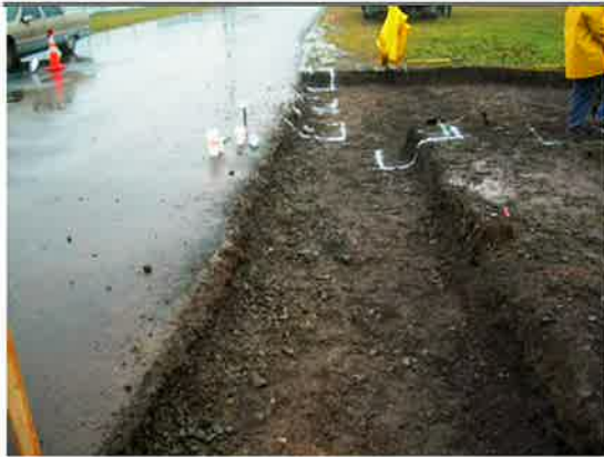
Picture 1: Sidewalk excavation and bollard layout
