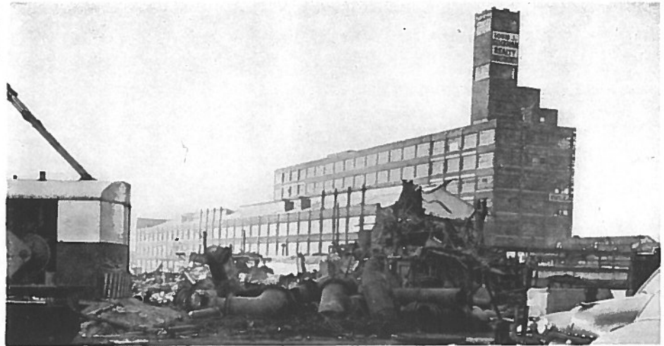
Only a pile of scrap remains at the site of the generator houses.
