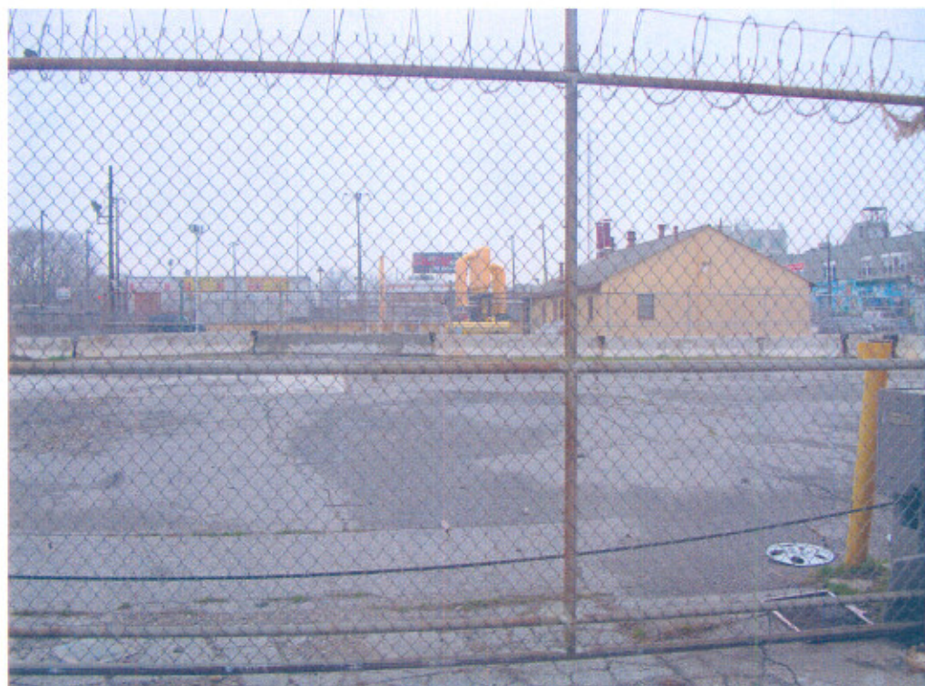
Photograph taken on April 2, 2007 of the southeastern portion of Holder Station B from 9 th Avenue.
