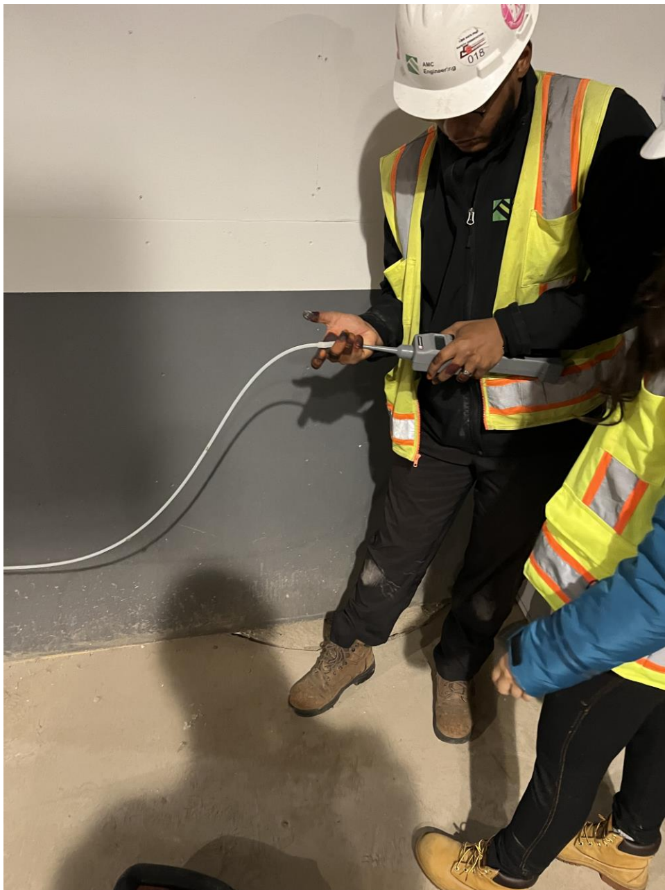
Observing Helium levels prior to Helium application.
