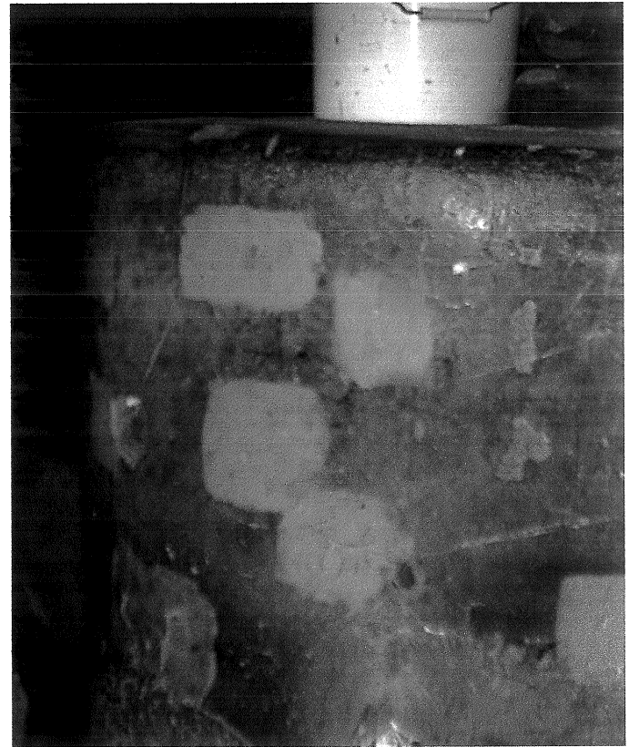
Suspect asbestos material covering boiler.
