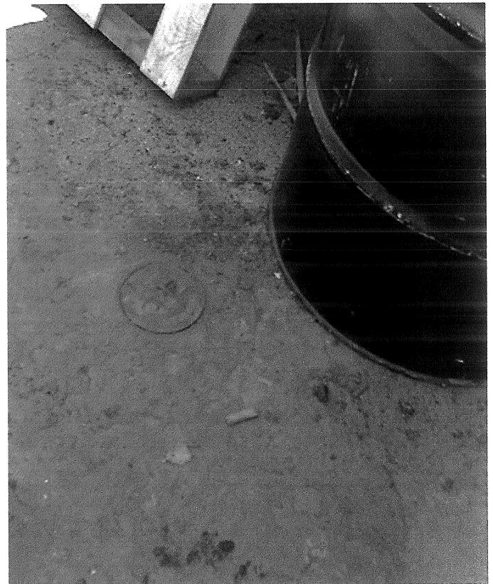
One of seventeen fill ports for USTs.
