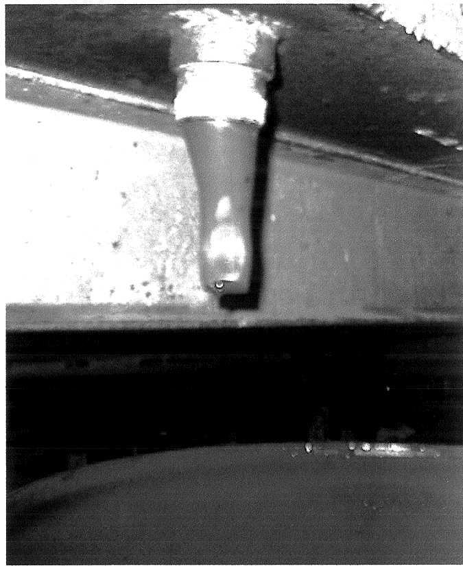
Active draining of AST for disposal.
