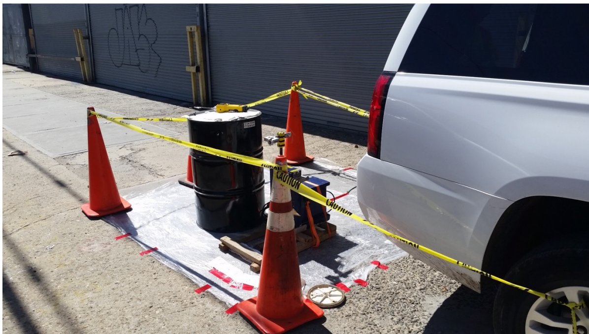
Photo 3: 9/14/15: Site Setup for DNAPL removal at 315 Kingsland Ave
