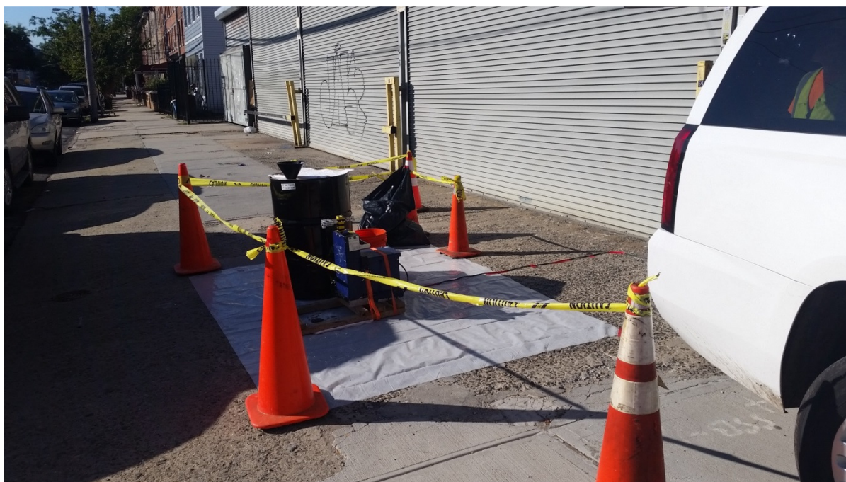
Photo 7: 9/15/15: Waterra pump set up for DNAPL removal at DEC-136.
