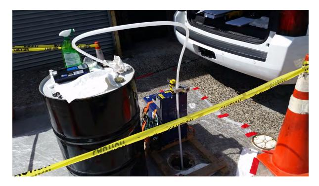
**Photo 6:** Waterra pump and drum set up for DNAPL removal at DEC-136 (Typical).
