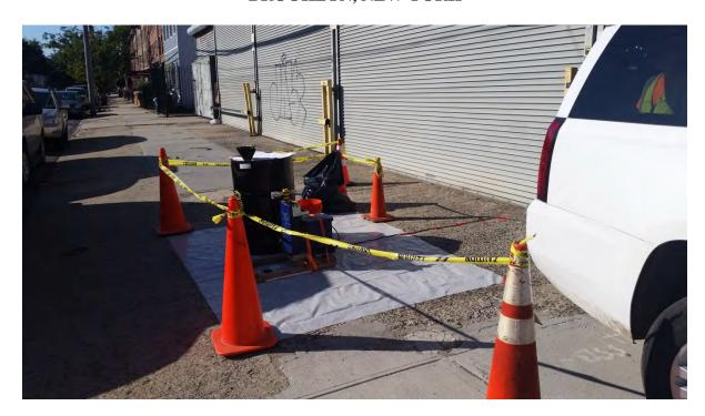
**Photo 7:** Waterra pump set up for DNAPL removal at DEC-136 (Typical).
