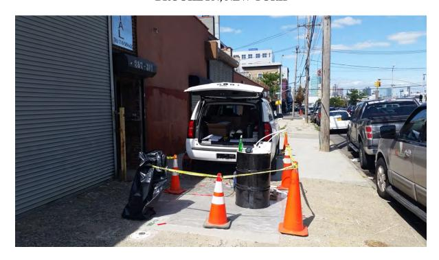
**Photo 5:** Site Setup for DNAPL removal at 315 Kingsland Ave. (Typical).
