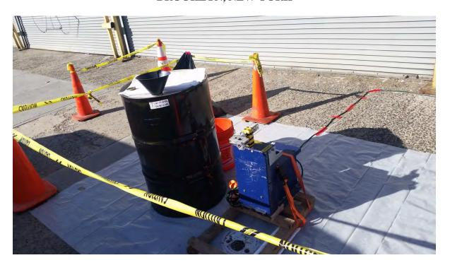
**Photo 9:** Waterra pump and drum set up for DNAPL removal at DEC-136 (Typical).
