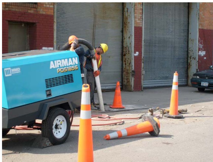
Photo 3: Example pre-clearing boring.
