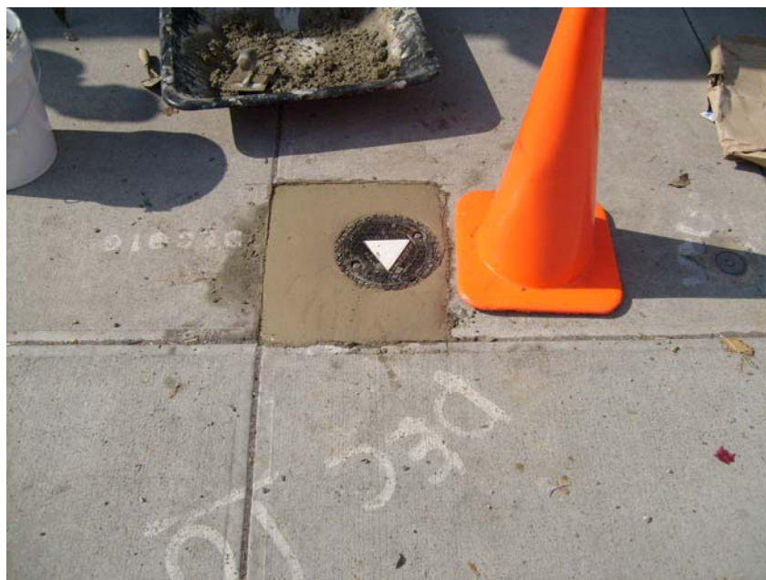
Photo 4: New flush-mount protective casing and well pad at DEC-010.
