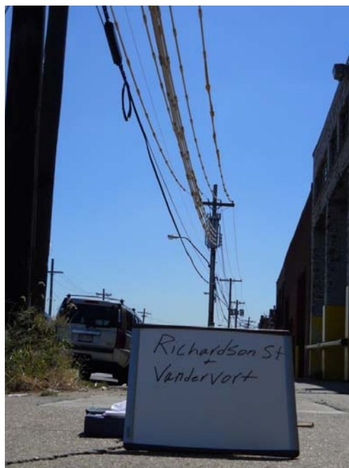
Photo 8: Insulating Jackets on Power Lines Near Richardson Street and Vandervoort Avenue.
