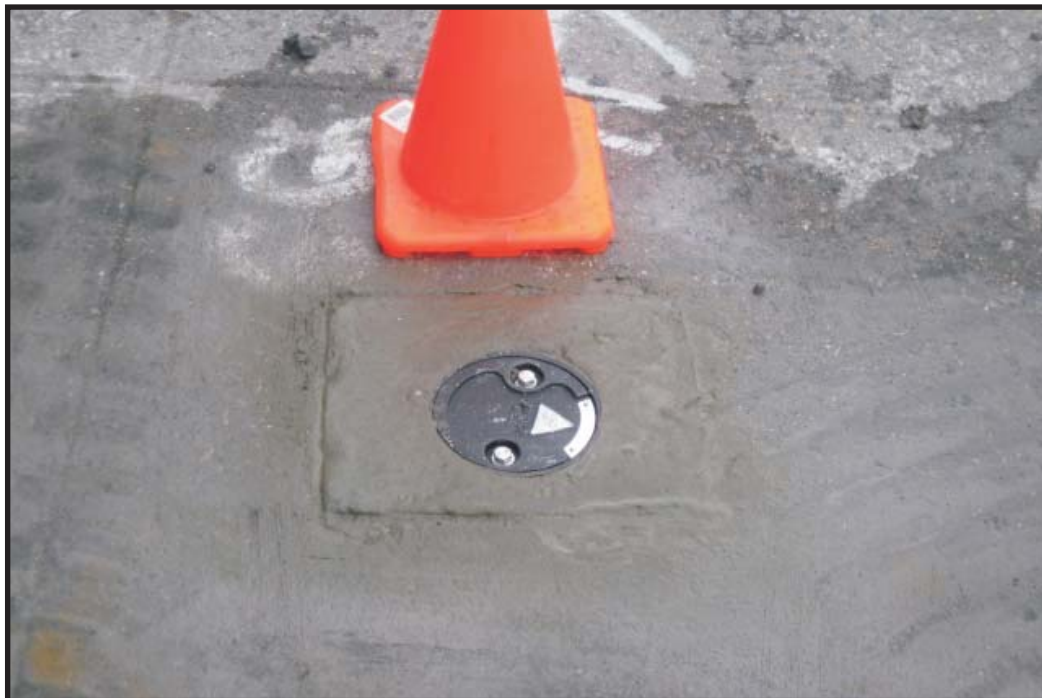
3/1/12: Completed soil-gas implant with 5-inch diameter flush-mount protective casing.
