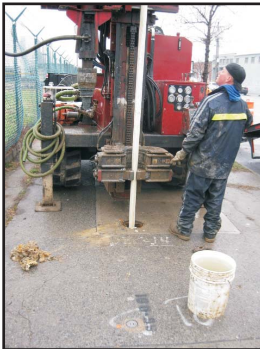
3/16/12: Removal of well string at DEC-014 during well decommissioning.
