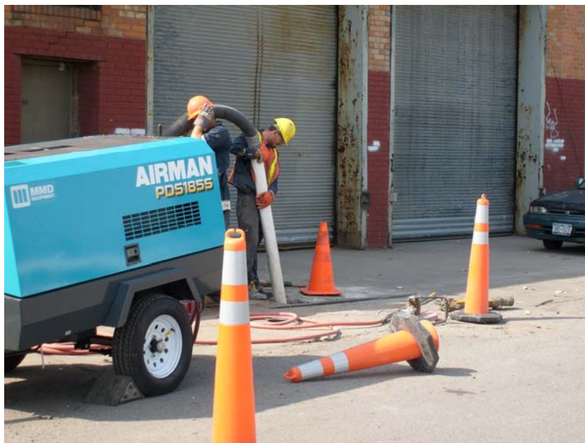
Photo 3: Example pre-clearing boring.
