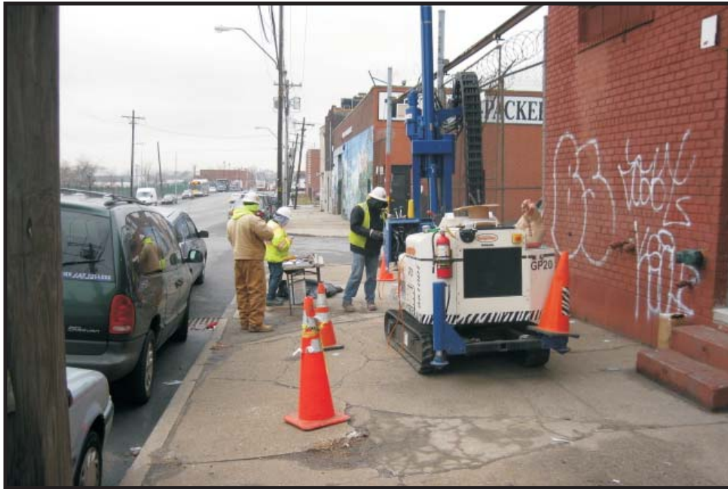
3/1/12: Advancement of soil boring at SG-119 prior to installation of soil-gas implant.
