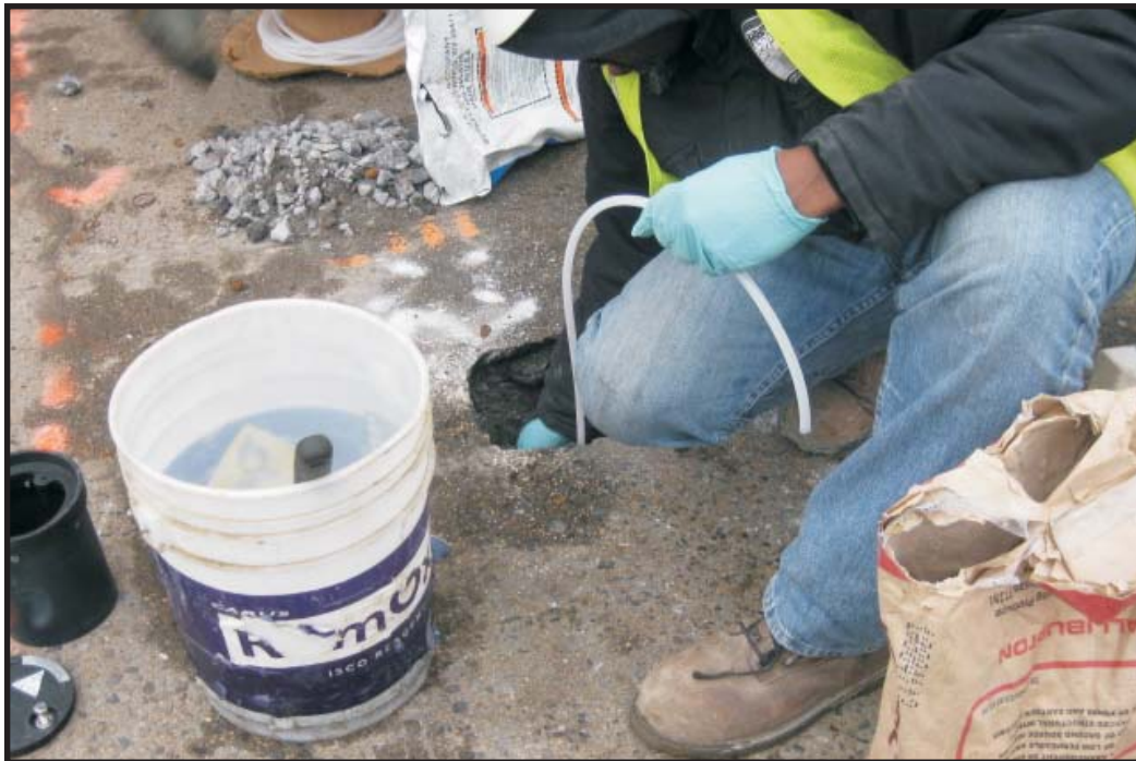
3/1/12: Installation of soil-gas implant at SG-119.
