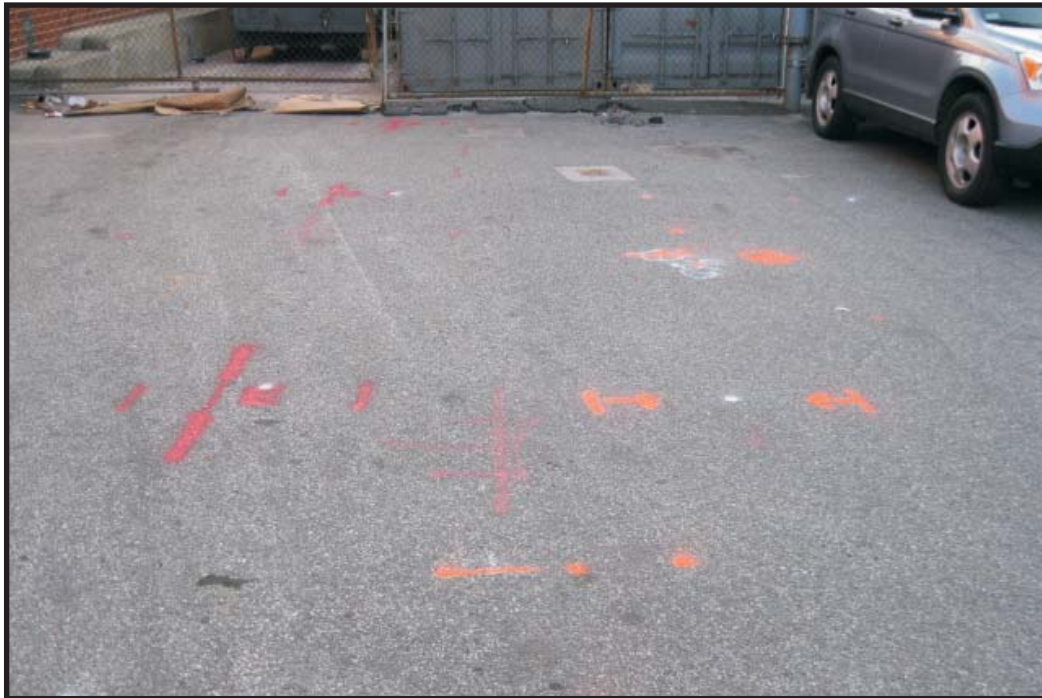
2/27/12: Example of geophysical utility mark outs around DEC-046D location.
