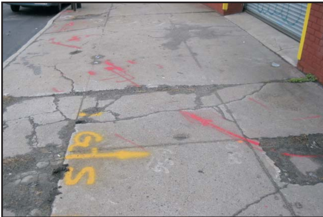
2/27/12: Example of geophysical utility mark outs around SG-116 location.
