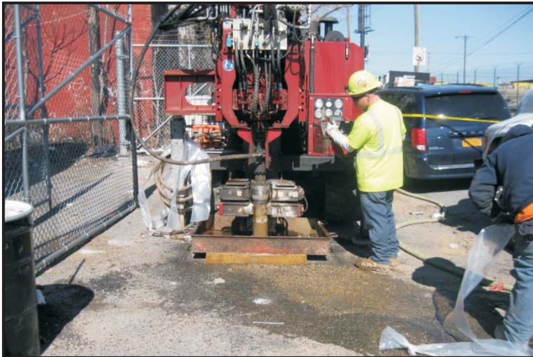
2/28/12: Sonic Drilling at DEC-088D.
