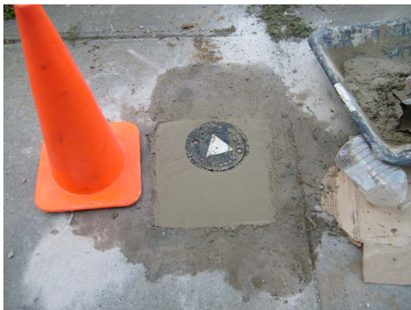
Photo 5: New flush-mount protective casing and well pad at DEC-031D.
