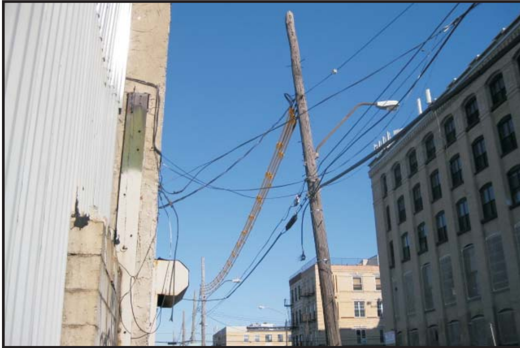
2/27/12: Photograph of overhead wires jacketed by Con Ed near DEC-011D.
