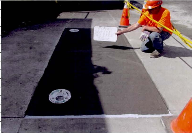
5/6/2014 - Completed flag at DEC-111 and DEC-111D
