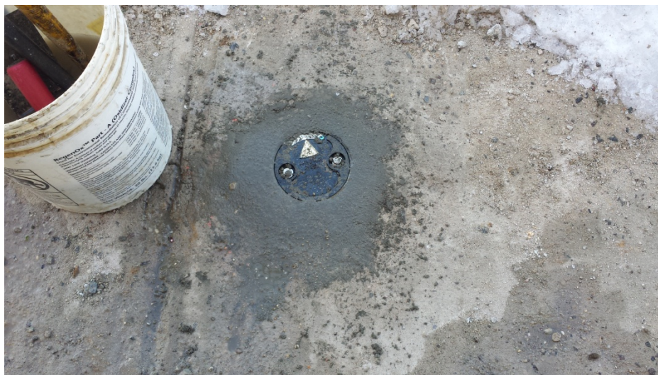
Photo 2: 2/7/14: SG-195 recently installed.
