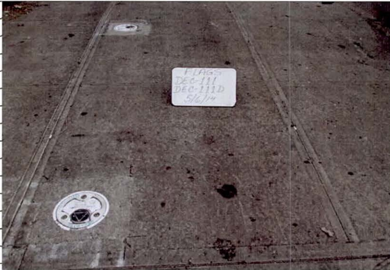
5/6/2014 - Flag at DEC-111 and DEC-111D prior to replacement
