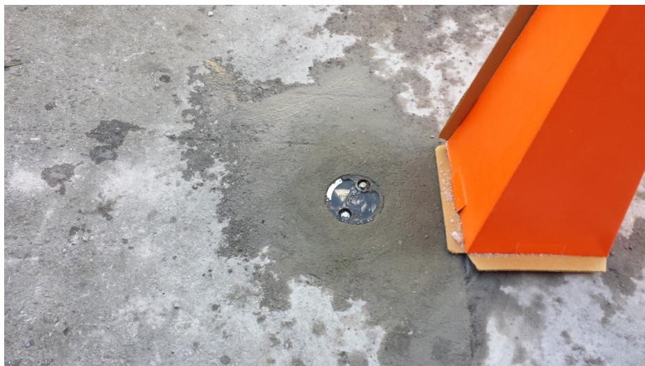
Photo 5: 2/7/14: SG-199 recently installed.
