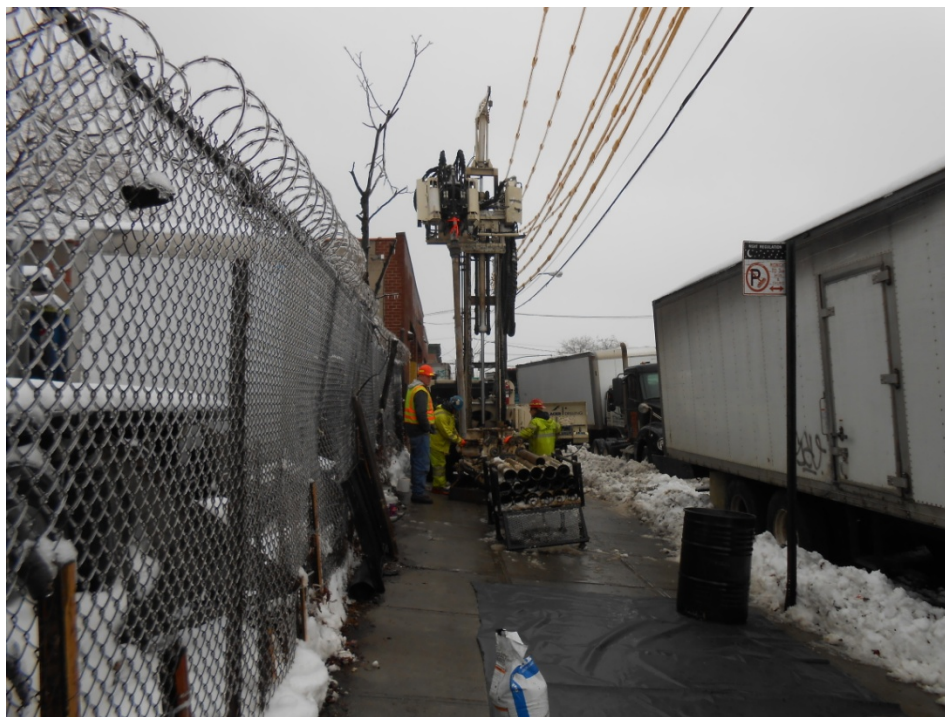
Photo 1: 2/5/14: Installation of DEC-111 and DEC-111D.
