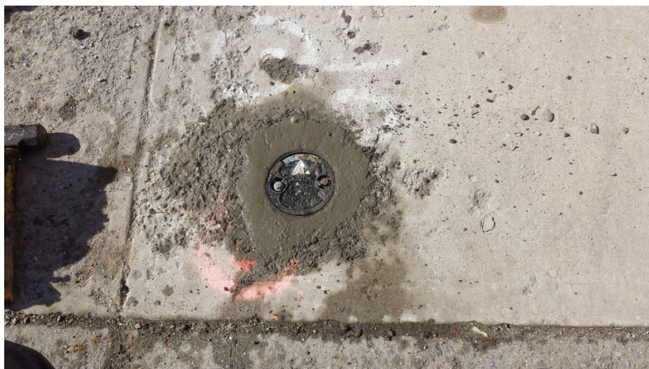
Photo 4: 2/7/14: SG-197 recently installed.
