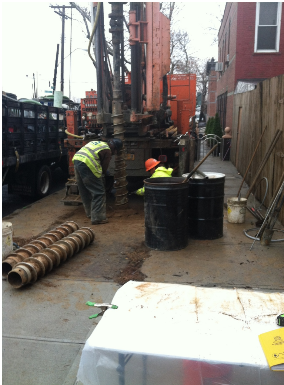
Photo 13: 12/13/13: Installation of DEC-006TC.
