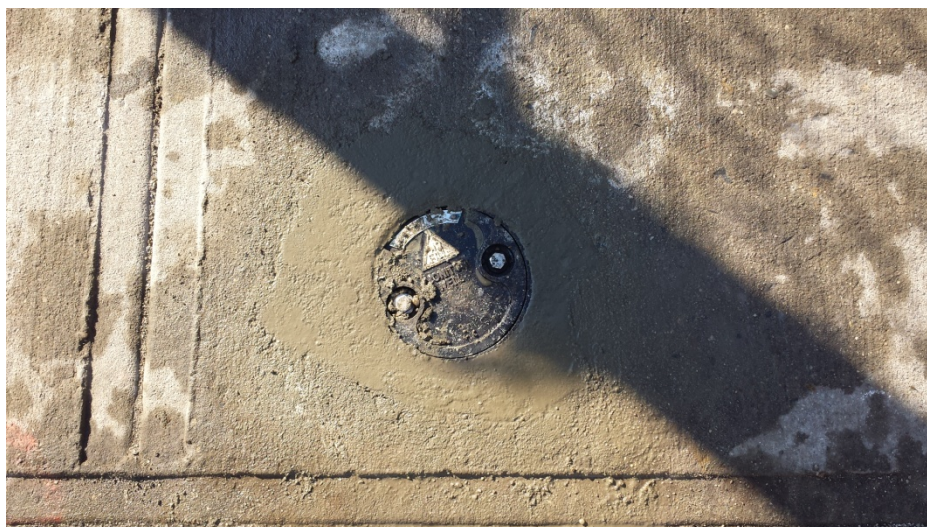
Photo 6: 2/7/14: SG-200 recently installed.
