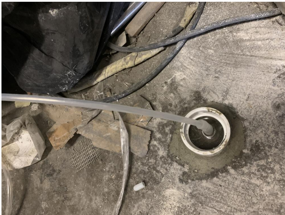
Photo 5: View of seal integrity test using a water dam at sub-slab soil vapor screening point ACME-SSVS-48 during purging process (12/21/2020)
