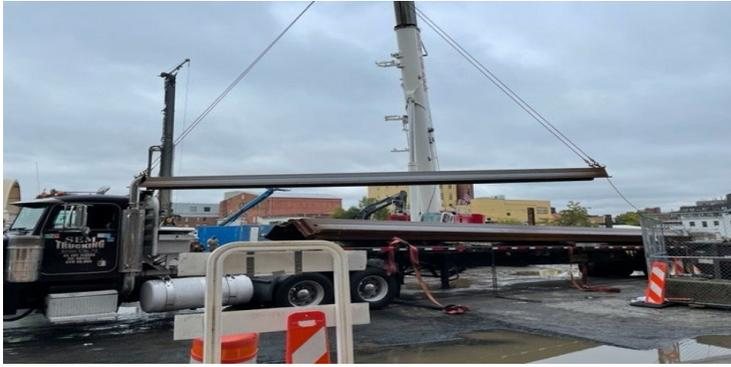
**Figure 8: Delivery of sheeting for coffer dam at DSNY Salt Lot**
