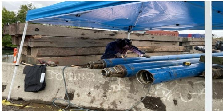
**Figure 7: Welding of centralizers on drill steel at DSNY Salt Lot**
