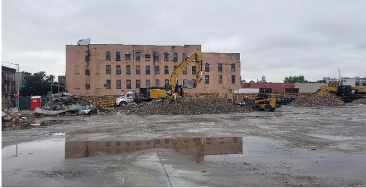
**Figure 5: Loading debris into dumpsters at 270 Nevins St.**
