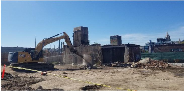
**Figure 2: Mechanical demolition at 517B Degraw St.**
