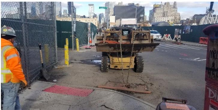
**Figure 4: Removing erosion control from catch basins around 270 Nevins St.**
