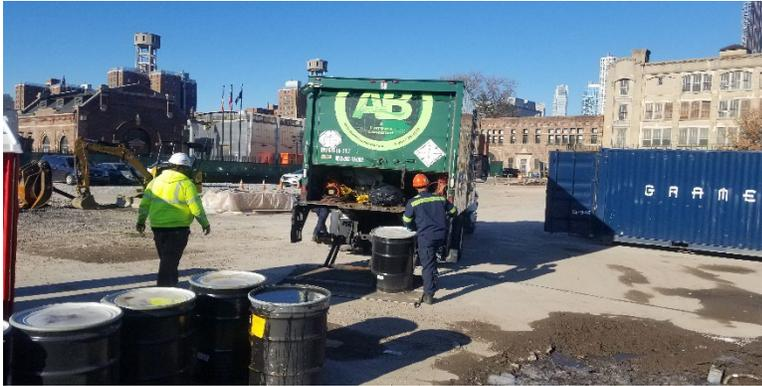
**Figure 2: Removing drum with soil from UST bottom**
