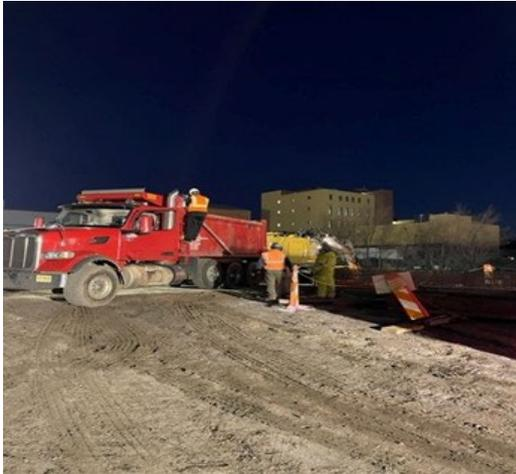
**Figure 8: Disposal of drilling spoils at DSNY Salt Lot**
