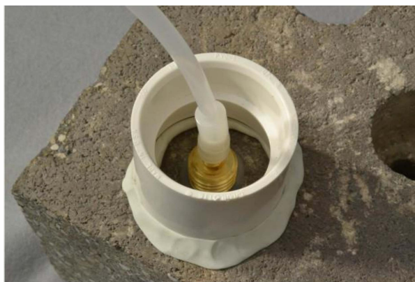
Figure 6. Water dam used for leak detection
