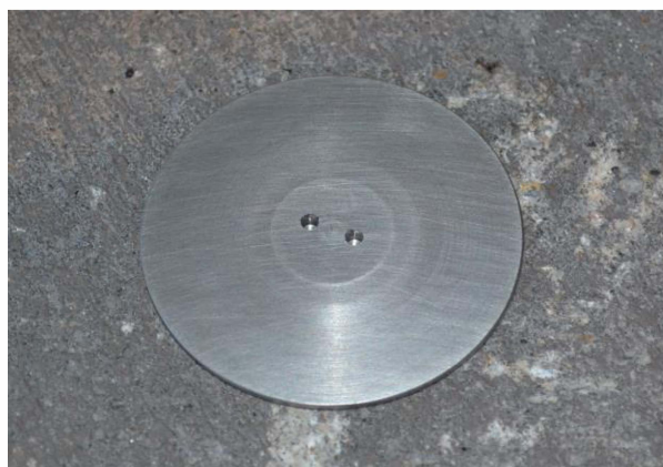
Figure 4. Secure Cover Installed
