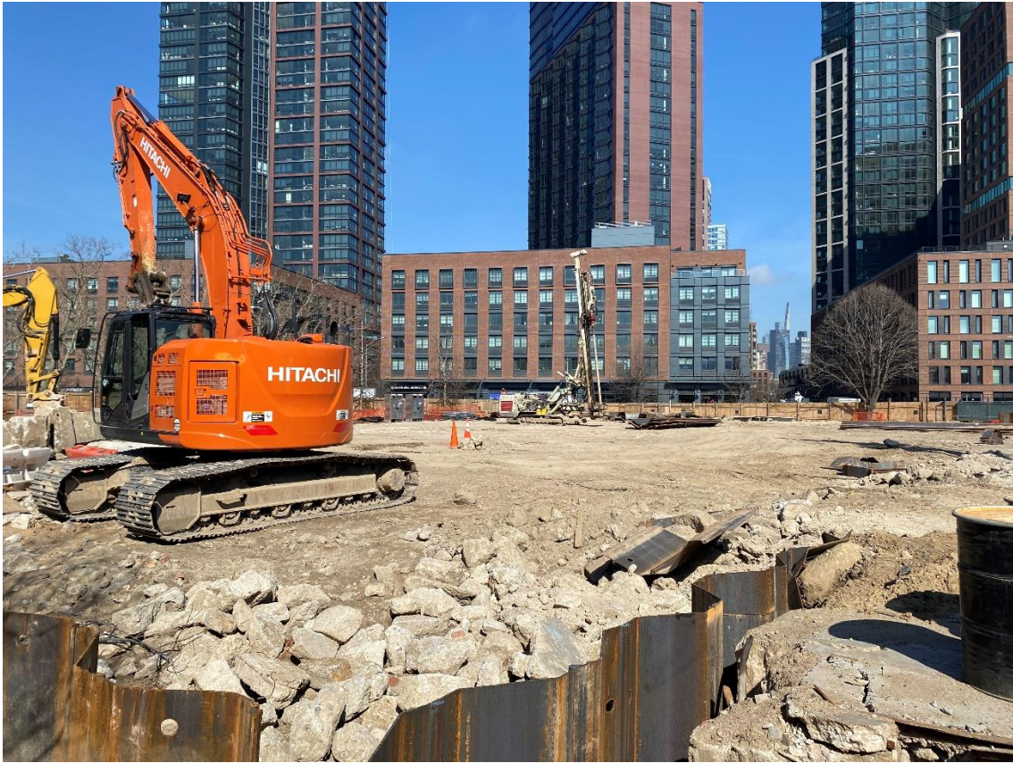
Photo 1: View of site, facing northwest.
