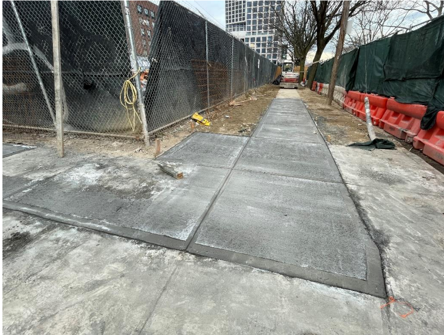
Photo 1: View of OU-2 work area facing west.
