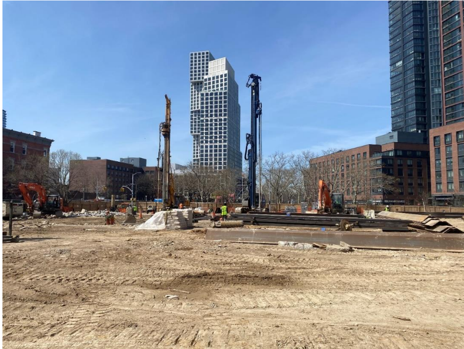
Photo 1: View of site conditions, facing west.
