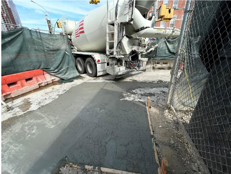
Photo 1: View of concrete pour at OU-2 work area facing east.
