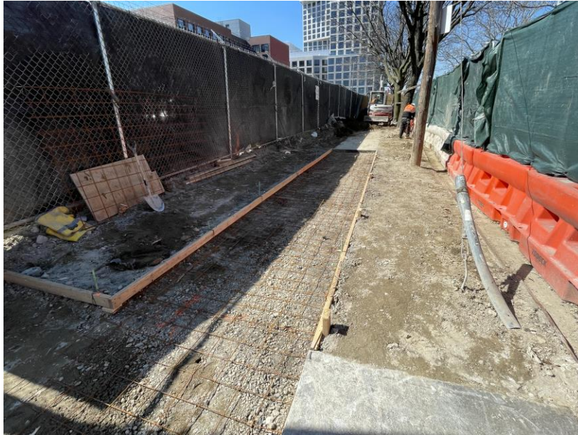
Photo 1: View of OU-2 work area facing west.
