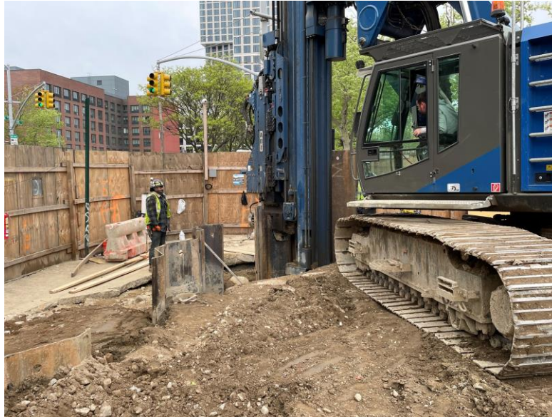
Photo 1: View of sheet pile installation, facing west.
