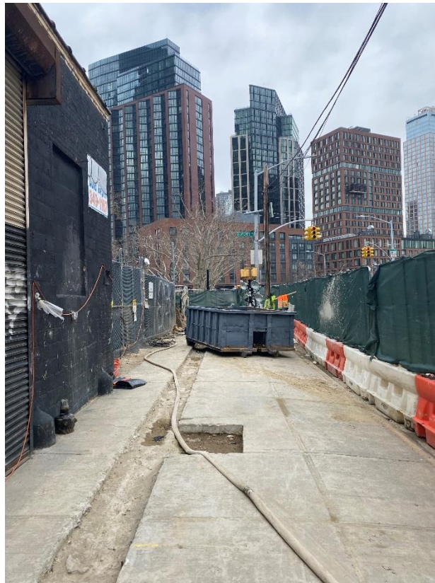
Photo 2: View of OU-2 work area facing northwest.
