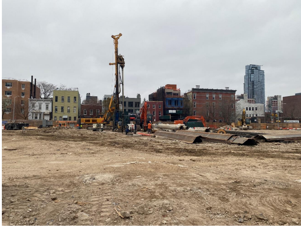
Photo 1: View of site conditions, facing south.
