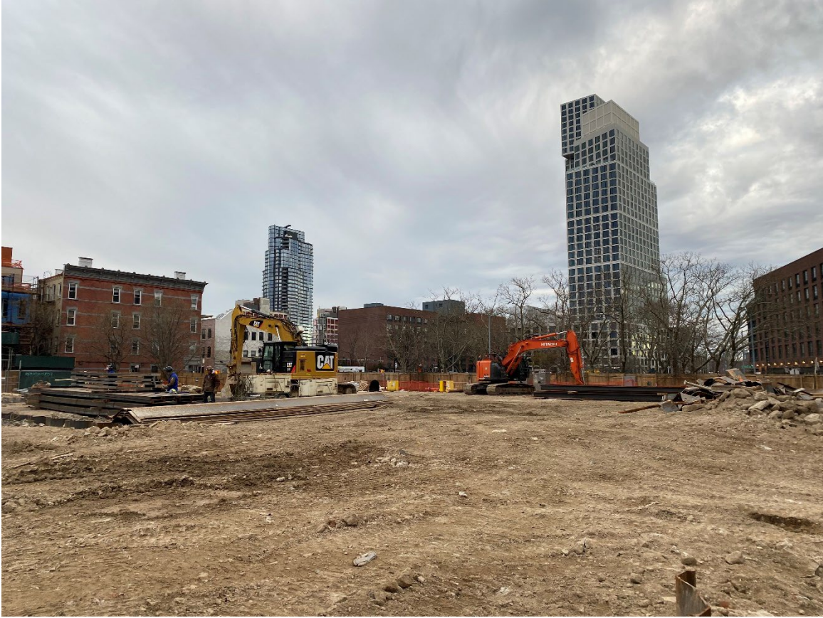
Photo 1: View of site conditions, facing southwest.
