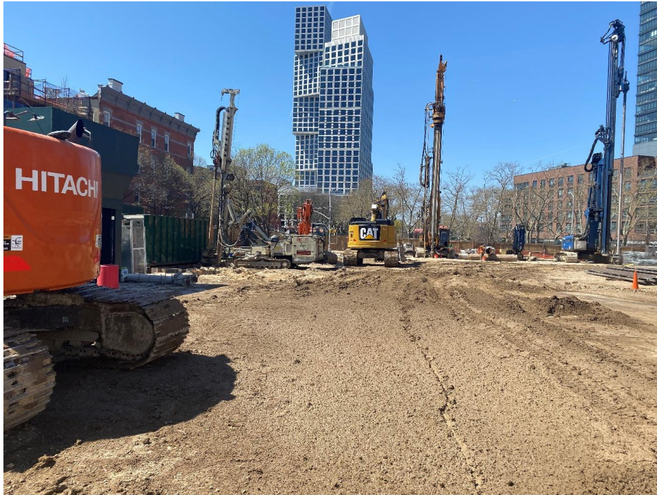
Photo 1: View of site conditions, facing west.
