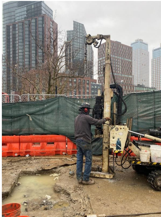
Photo 1: View of OU-2 monitoring well installation facing north.
