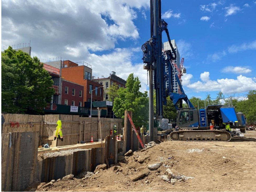
Photo 1: View of sheet pile installation, facing southwest.
