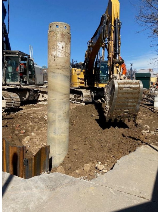
Photo 1: View of obstruction clearing for sheet pile installation, facing northeast.
