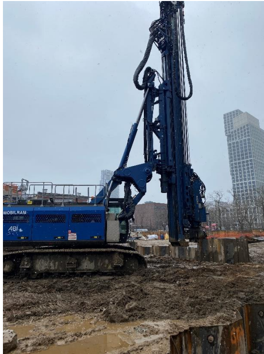
Photo 1: View of OU-1 sheet pile wall installation facing southwest.
