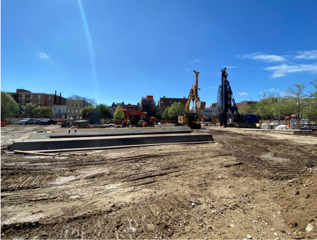
Photo 1: View of site conditions, facing southwest.
