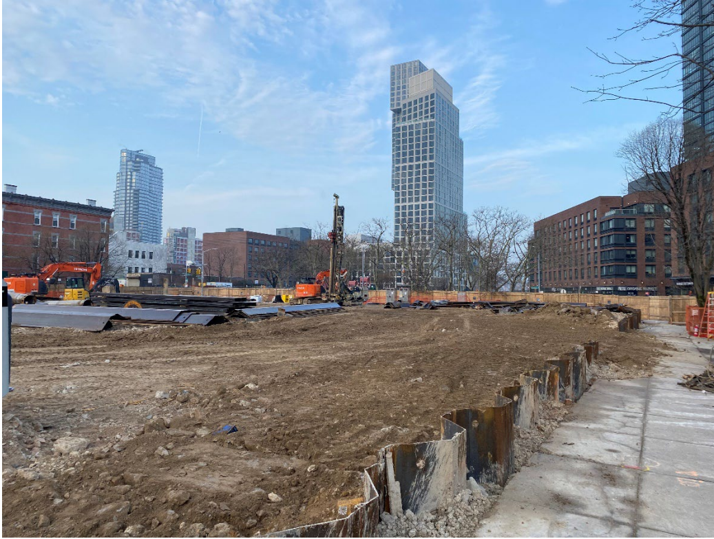
Photo 1: View of site conditions, facing southwest.
