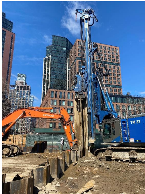
Photo 2: Alternate view of OU-1 sheet pile wall installation facing west.
