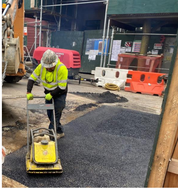
Photo 1: View of asphalt leveling over completed street excavation, facing south.
