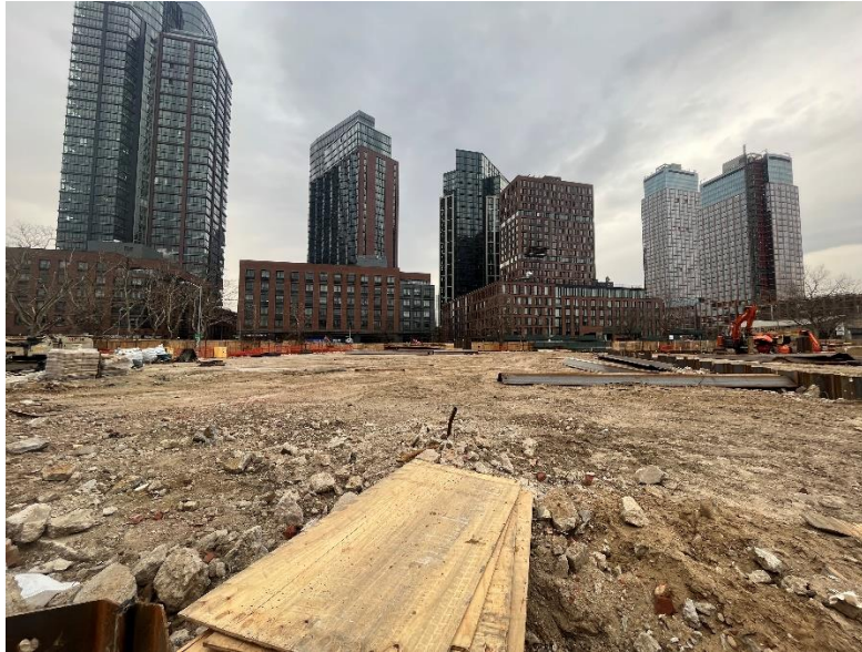
Photo 1: View of the site facing north.
