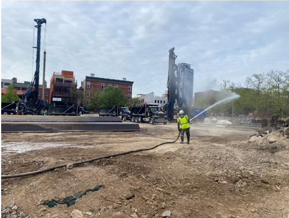
Photo 1: View of site conditions, facing southwest.
