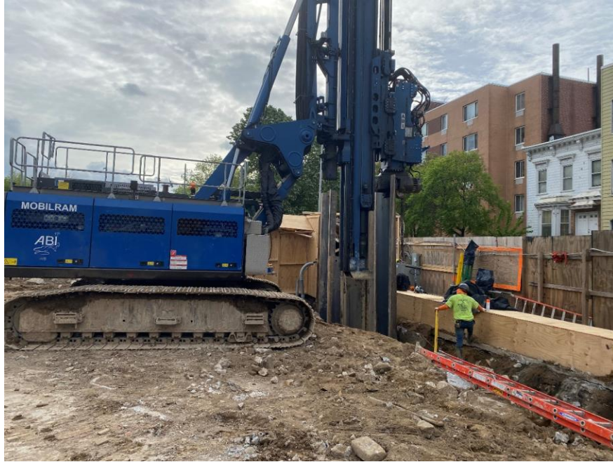
Photo 1: View of sheet pile installation, facing southeast.
