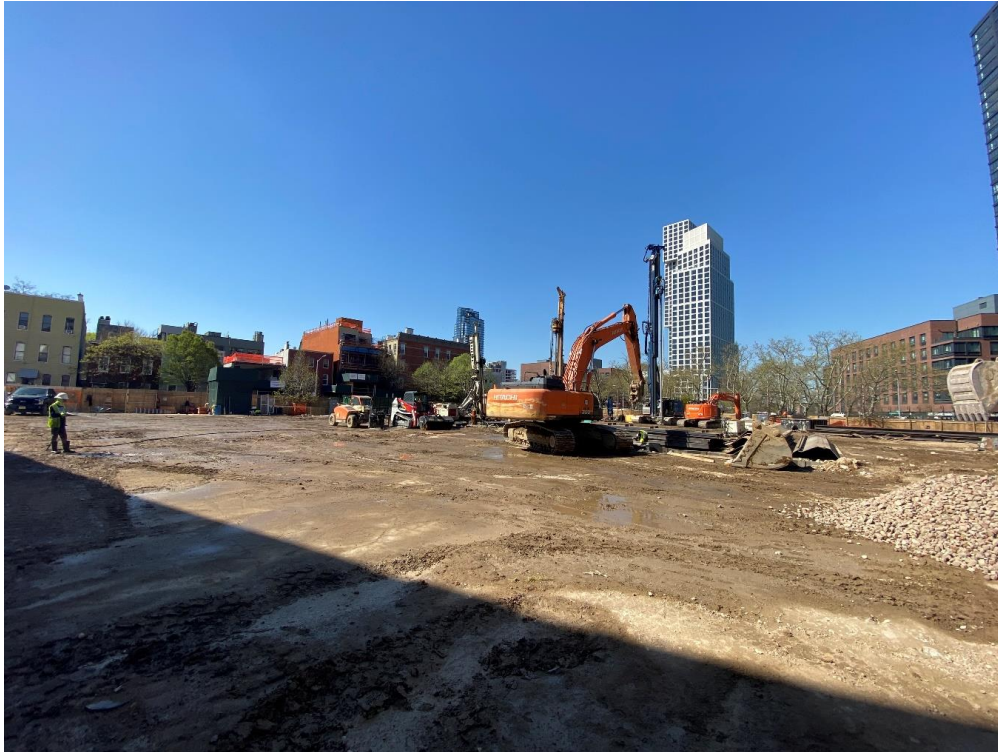
Photo 1: View of site conditions, facing southwest.
