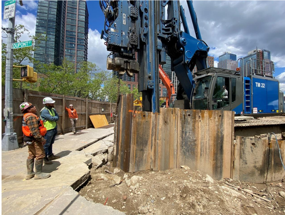
Photo 1: View of sheet pile installation, facing west.
