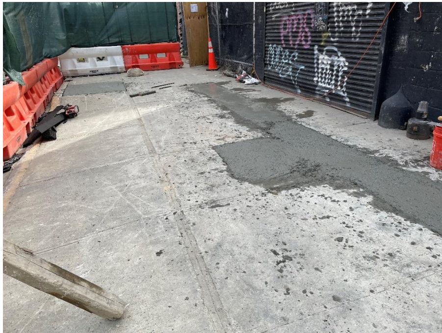
Photo 2: Alternate view of concrete pour at OU-2 work area facing south.
