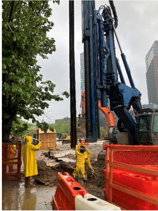
Photo 1: View of sheet pile installation, facing northwest.
