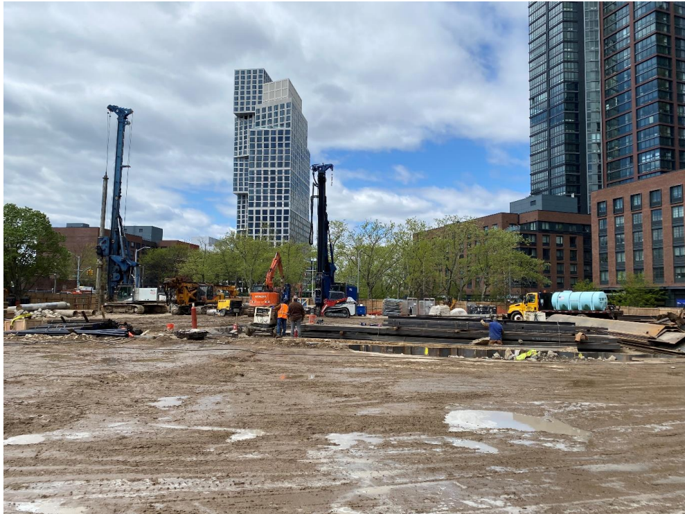
Photo 1: View of site conditions, facing west.
