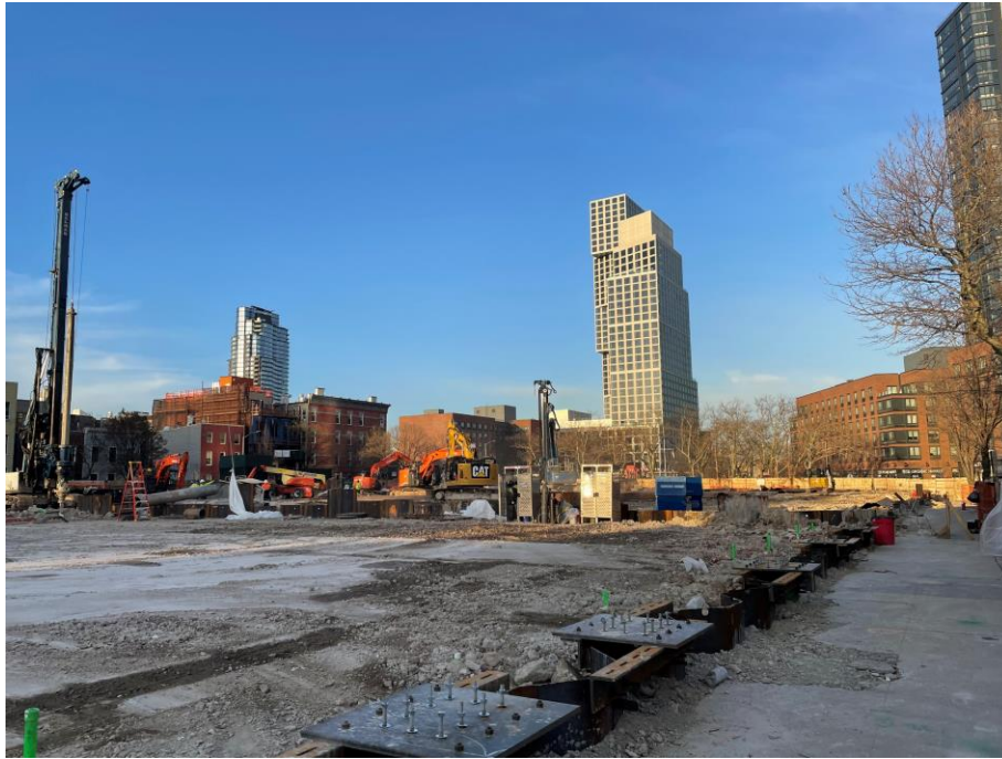
Photo 1: View of the site facing west.
