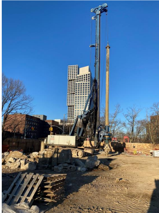
Photo 1: View of drill rig mobilized to clear obstructions for sheet pile installation.
