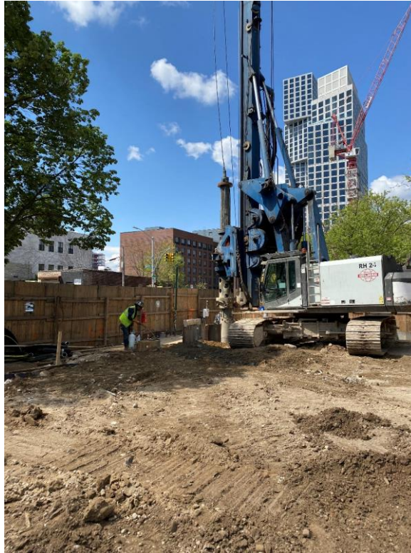
Photo 1: View of sheet pile installation, facing southwest.
