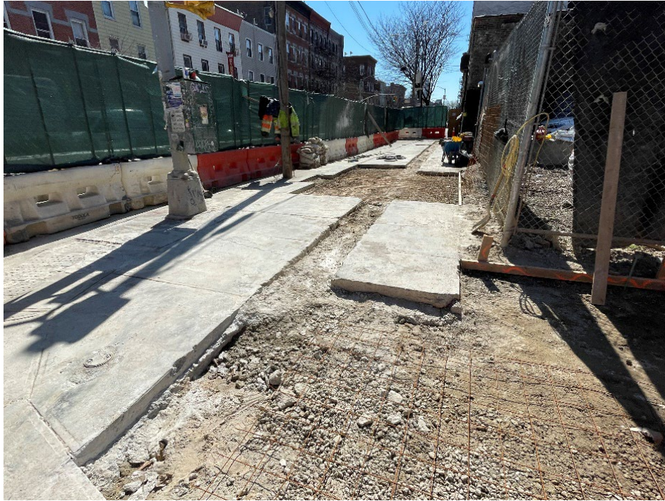
Photo 1: View of OU-2 work area facing south.
