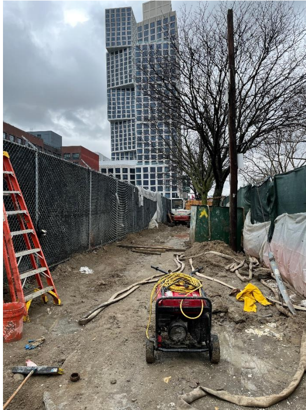
Photo 1: View of OU-2 work area facing west.
