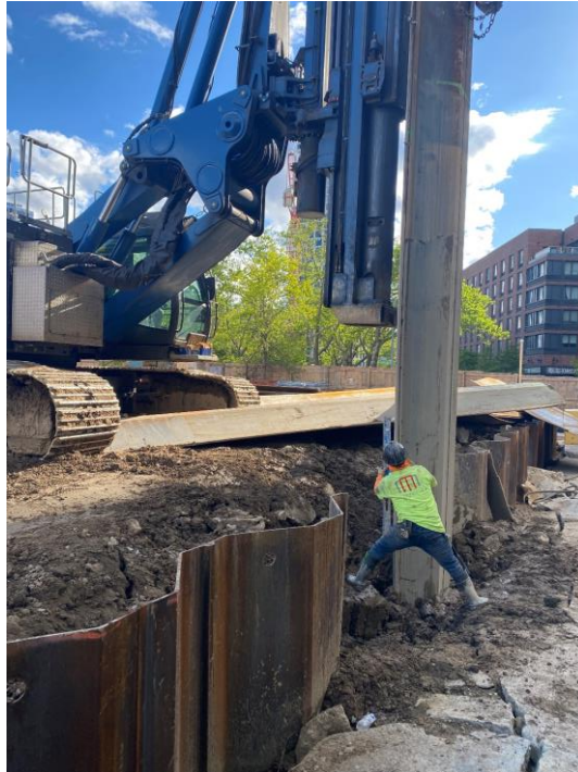
Photo 1: View of sheet pile installation, facing west.
