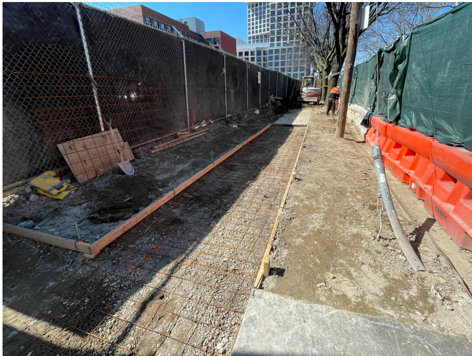
Photo 2: View of OU-2 work area facing west.
