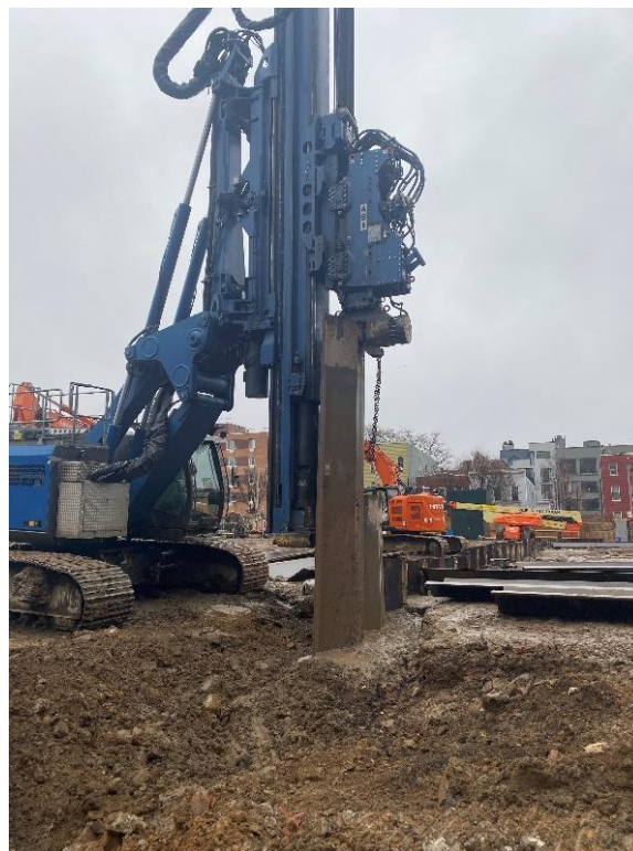
Photo 2: View of OU-1 sheet pile wall installation facing south.
