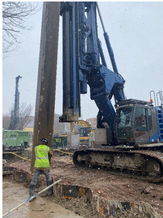
Photo 2: Alternative view of OU-1 sheet pile wall installation facing southeast.
