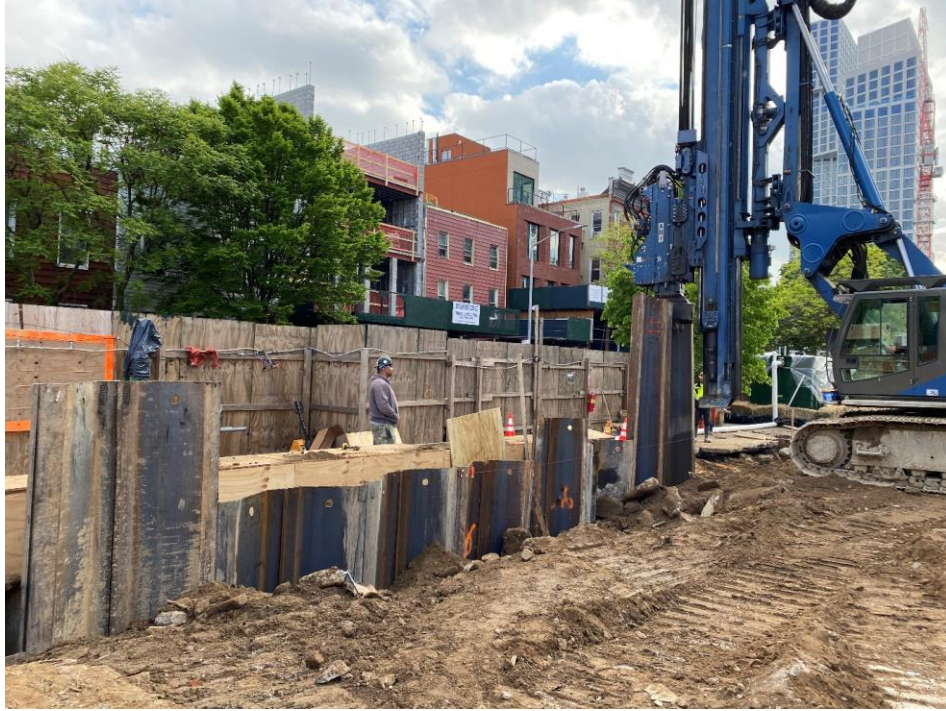
Photo 1: View of sheet pile installation, facing southwest.
