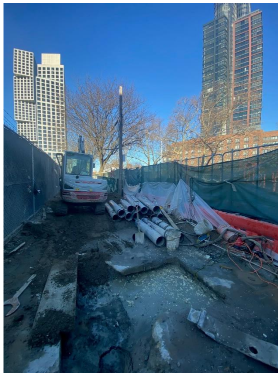
Photo 2: View of OU-2 work area facing northwest.
