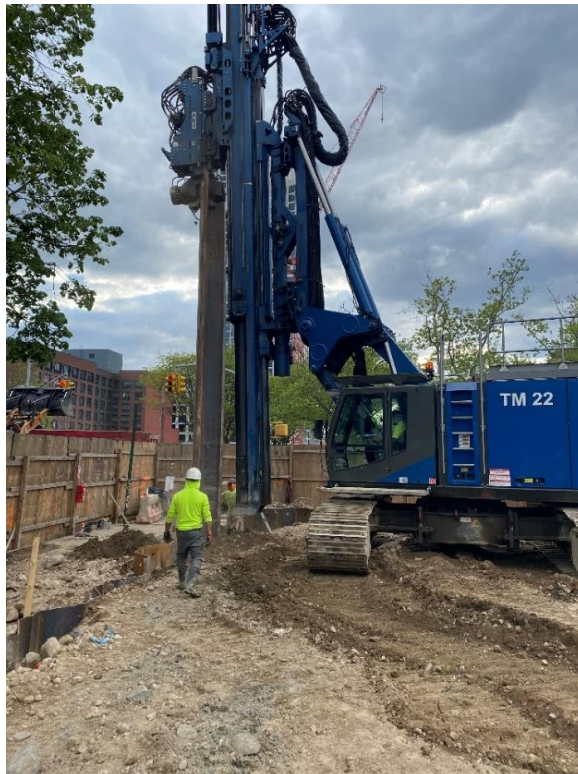
Photo 2: View of sheet pile installation, facing southwest.
