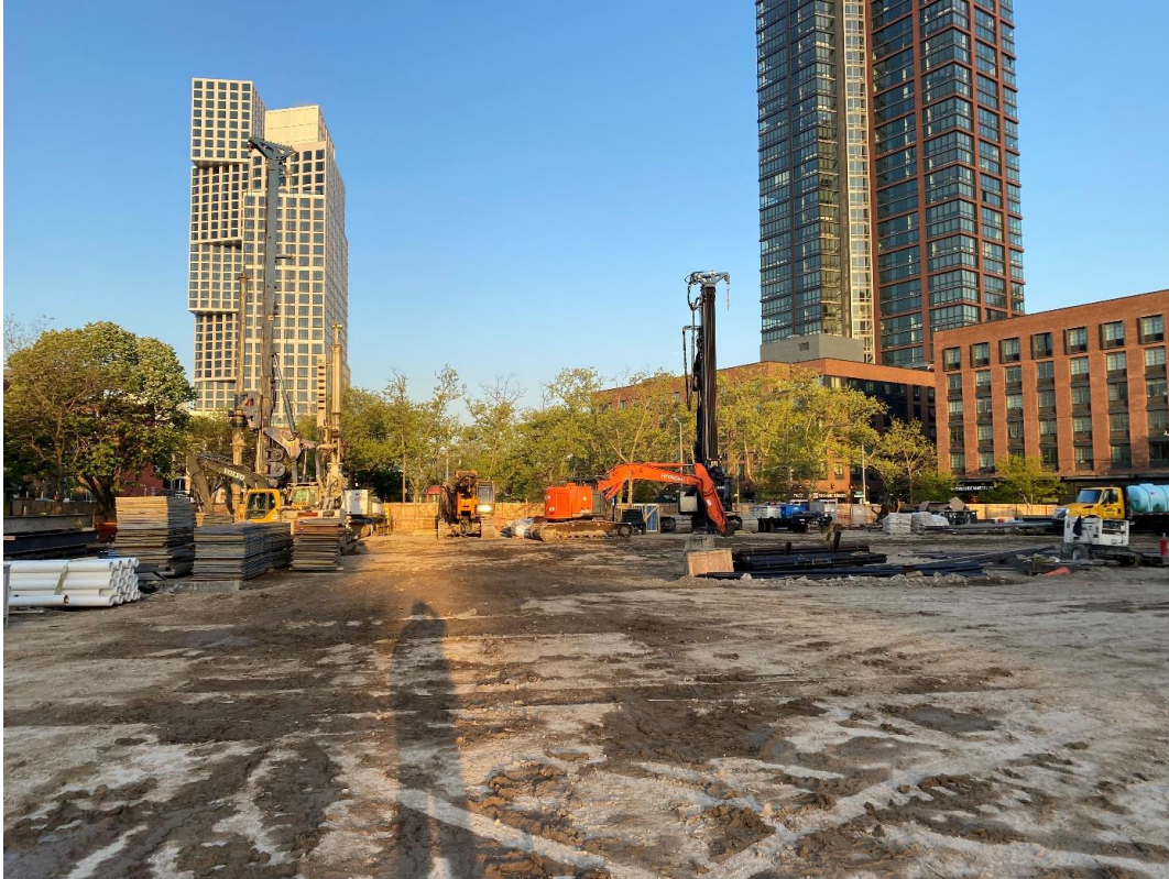
Photo 1: View of site conditions, facing west.
