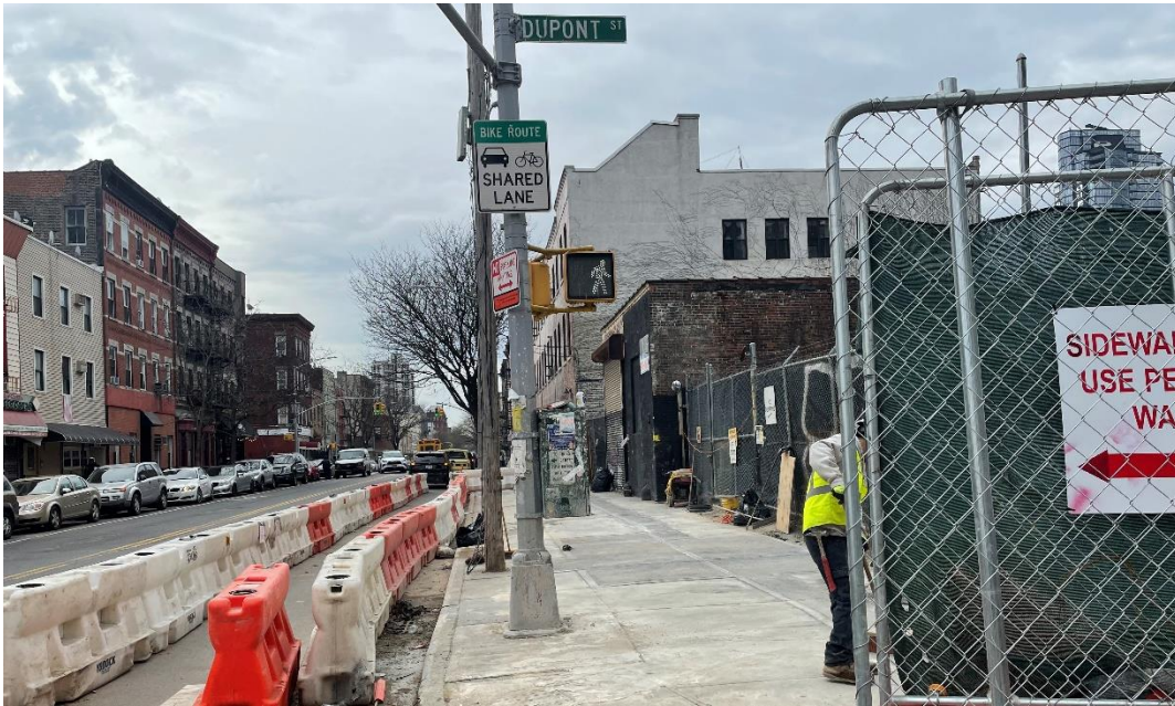
Photo 1: View of OU-2 restored sidewalk facing south.
