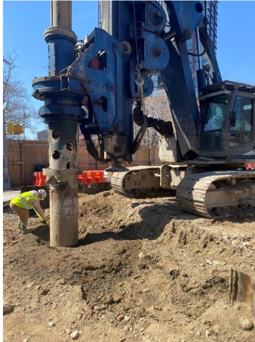
Photo 1: View of obstruction clearing for sheet pile installation, facing northwest.
