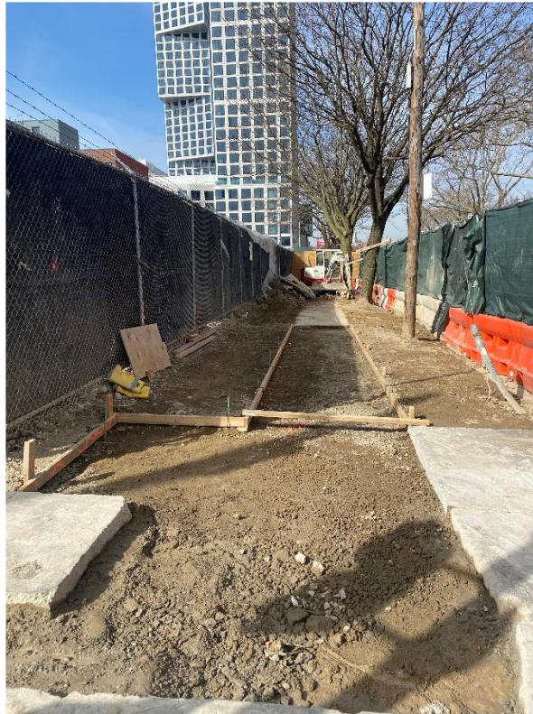
Photo 1: View of OU-2 sidewalk restoration formwork, facing west.
