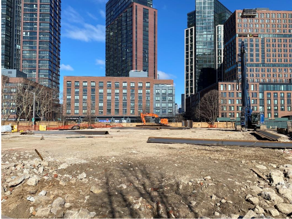
Photo 1: View of the site facing north.
