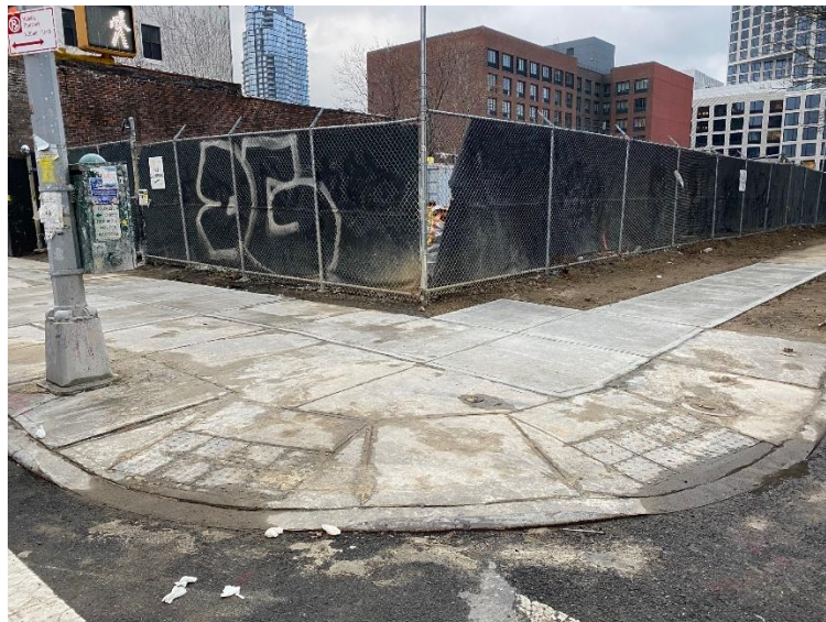
Photo 1: View of restored OU-2 sidewalk facing southwest.
