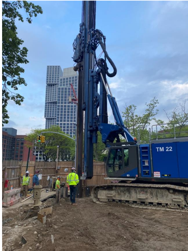
Photo 1: View of sheet pile installation, facing west.
