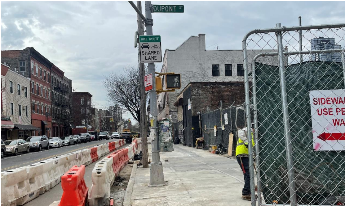
Photo 1: View of OU-2 work area restoration facing south.
