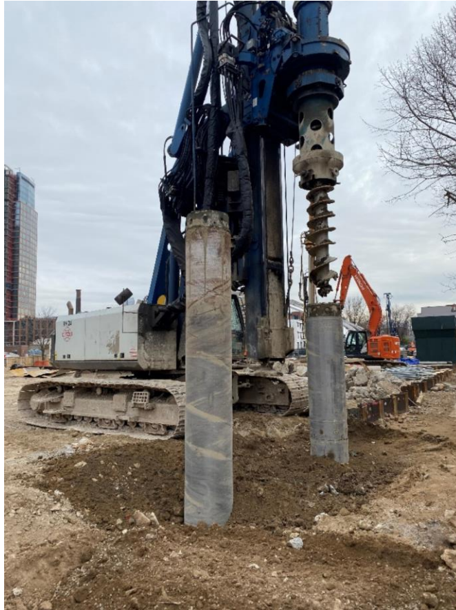
Photo 1: View of drill rig clearing obstructions for sheet pile installation, facing northeast.
