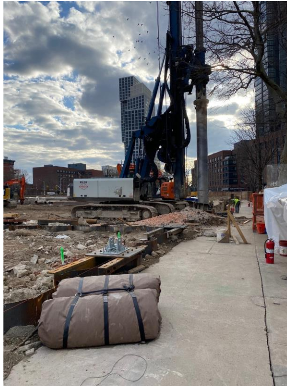
Photo 1: View of contractor drilling through sheet pile obstructions facing west.
