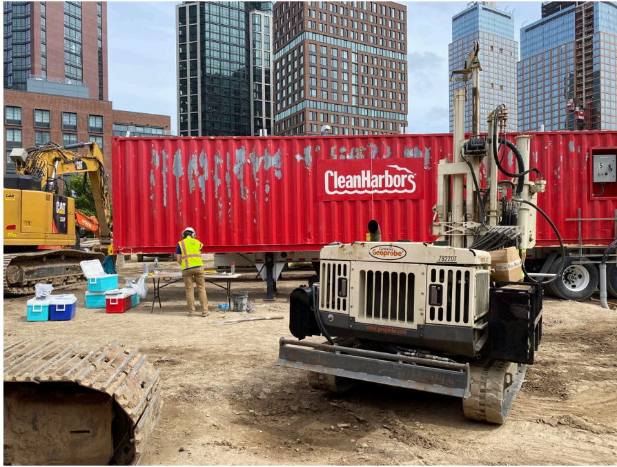
Photo 1: View of drilling for Supplemental Waste Characterization sampling.
