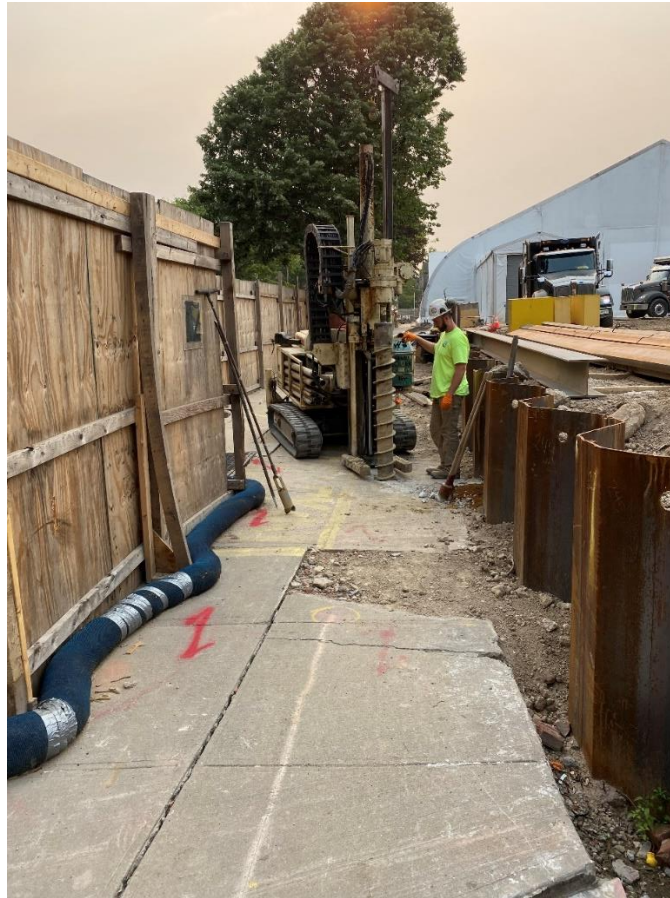
Photo 1: View of LNAPL recovery well installation, facing east.
