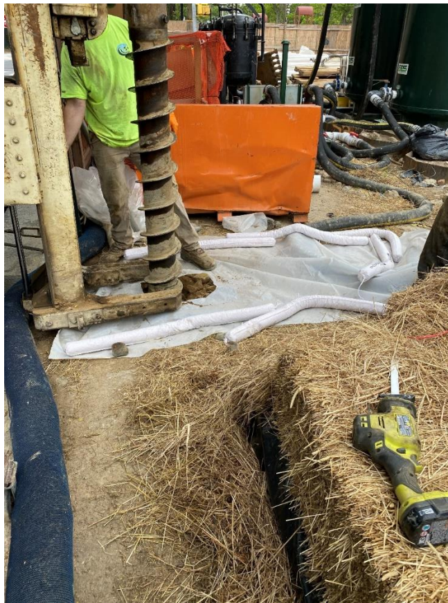
Photo 1: View of LNAPL recovery well installation, facing west.
