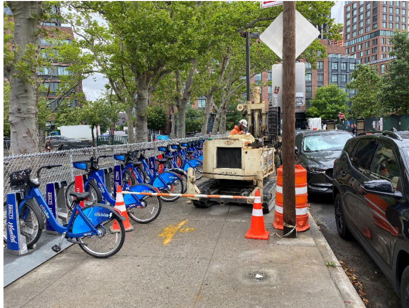
Photo 1: View of off-site LNAPL recovery well installation, facing north.
