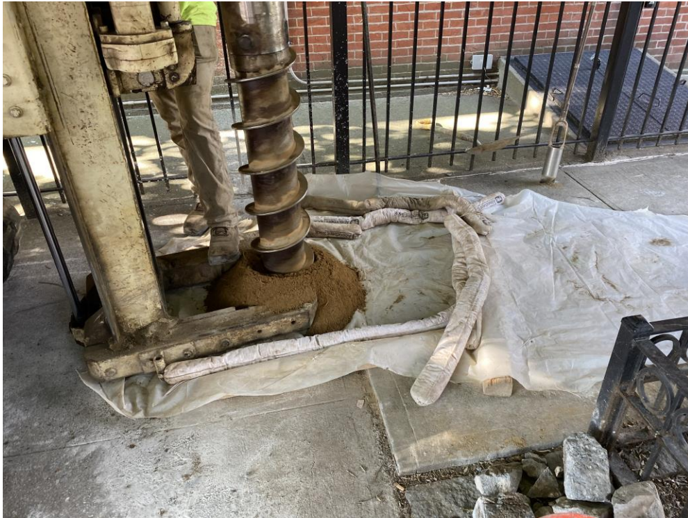
Photo 1: View of off-site LNAPL recovery well installation, facing south.
