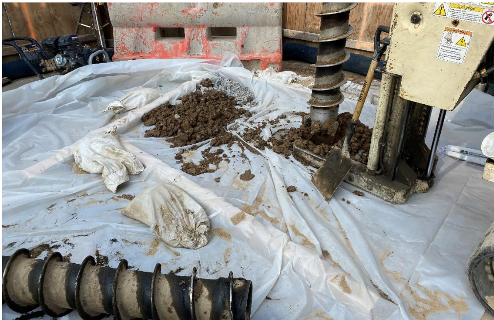
Photo 1: View of LNAPL recovery well installation, facing southwest.
