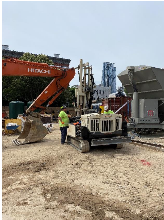
Photo 1: View of drilling for Supplemental Waste Characterization sampling.
