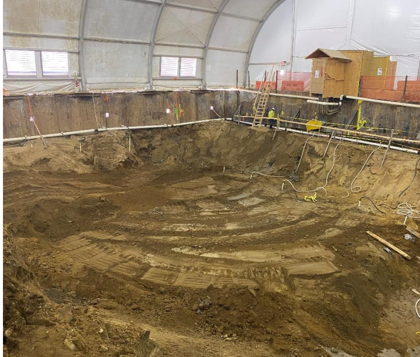
Photo 1: View of excavation and dewatering system within the enclosure.
