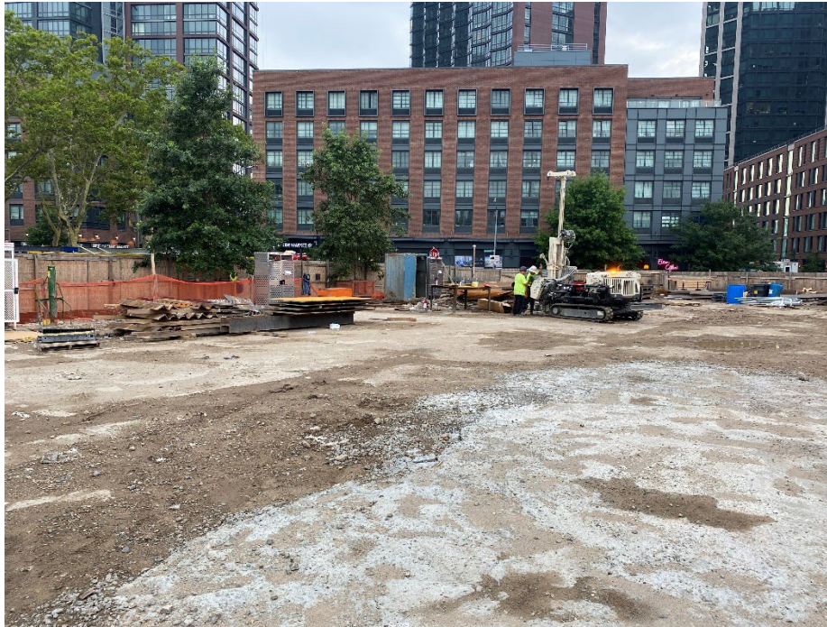
Photo 1: View of delineation boring installation, facing northeast.
