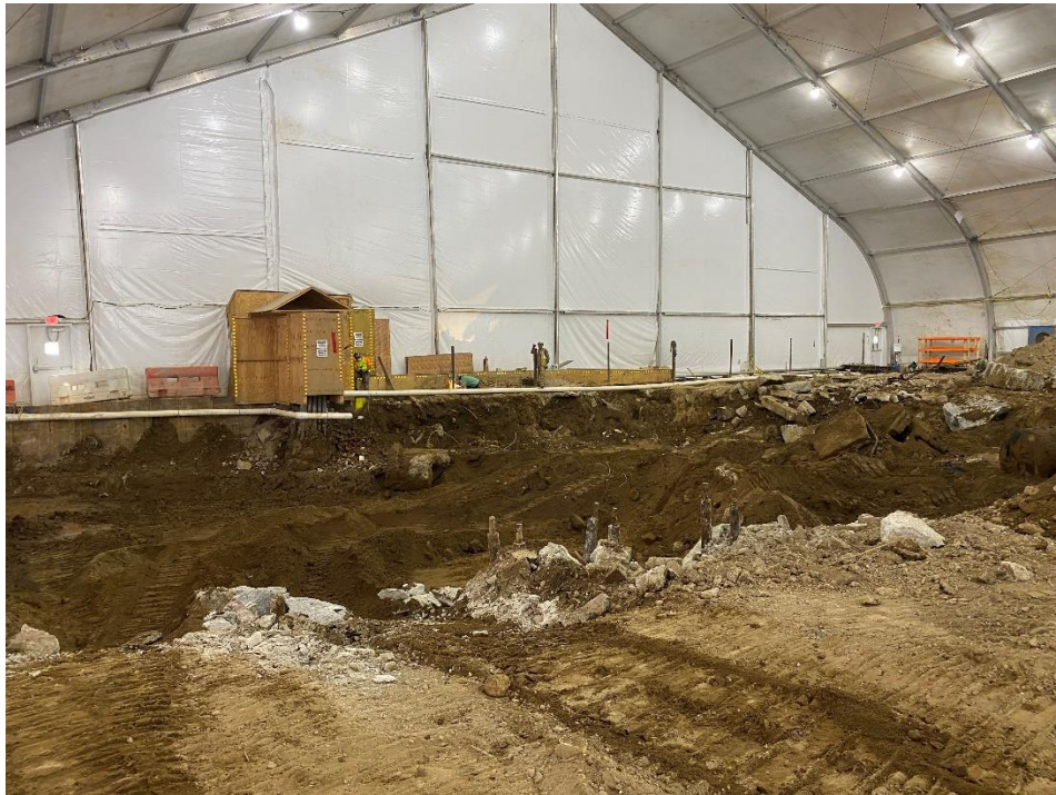
Photo 2: View of slab demolition and soil excavation within enclosure, facing southwest.
