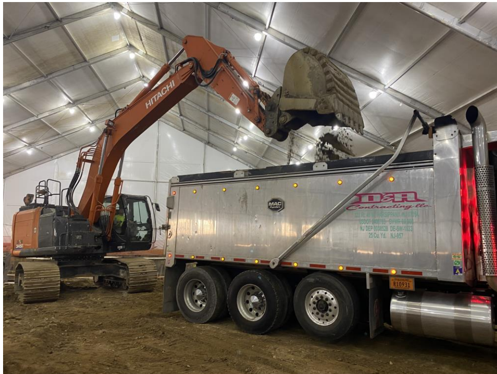
Photo 2: View of excavated soil loading within the enclosure.
