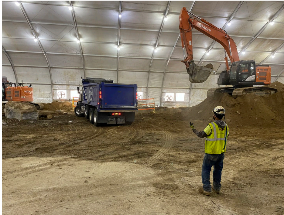
Photo 1: View of excavated soil loading within the enclosure, facing east.
