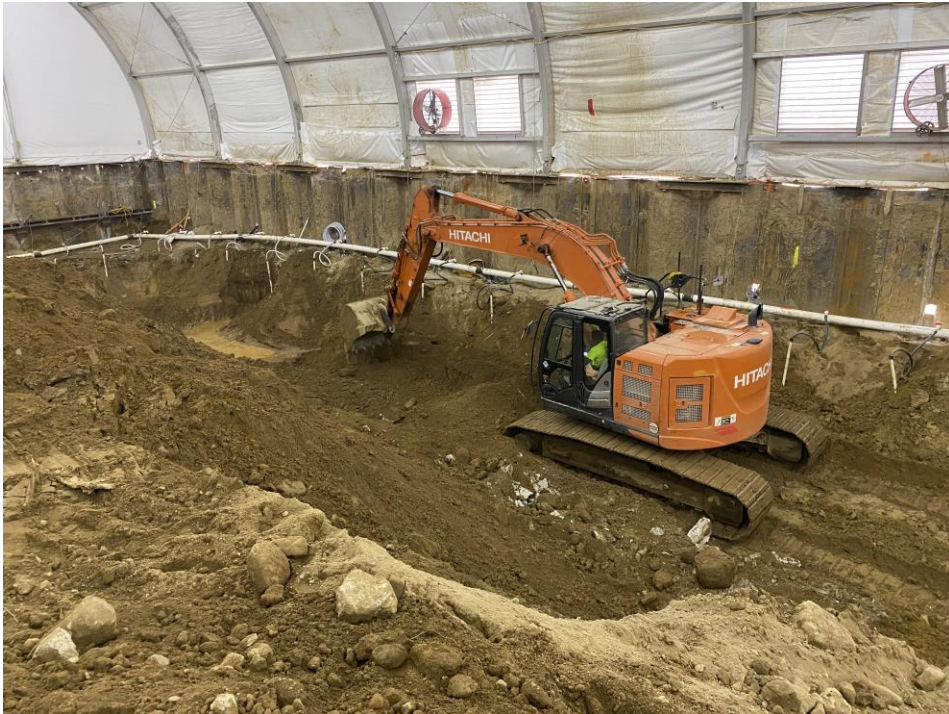
Photo 2: View of excavation and dewatering system within the enclosure.
