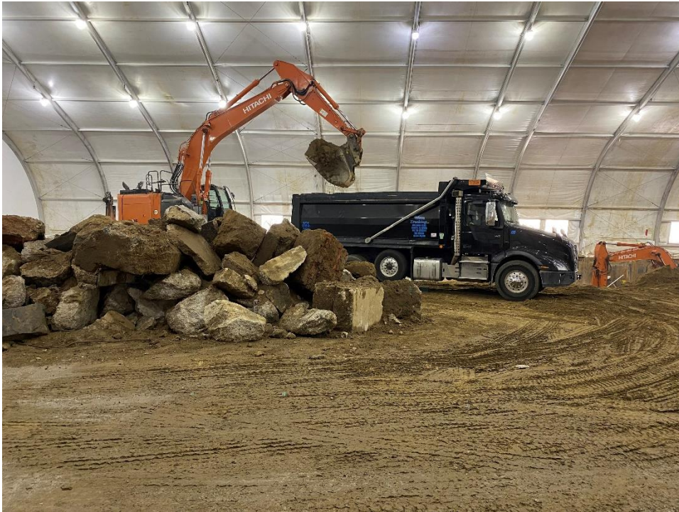
Photo 2: View of soil loading inside the enclosure facing east.
