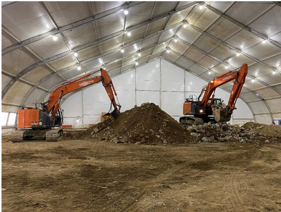
Photo 2: View of slab demolition and soil stockpile within enclosure, facing south.
