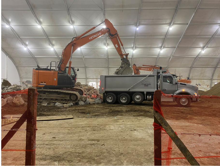
Photo 1: View of C&D debris material loading within the enclosure, facing east.
