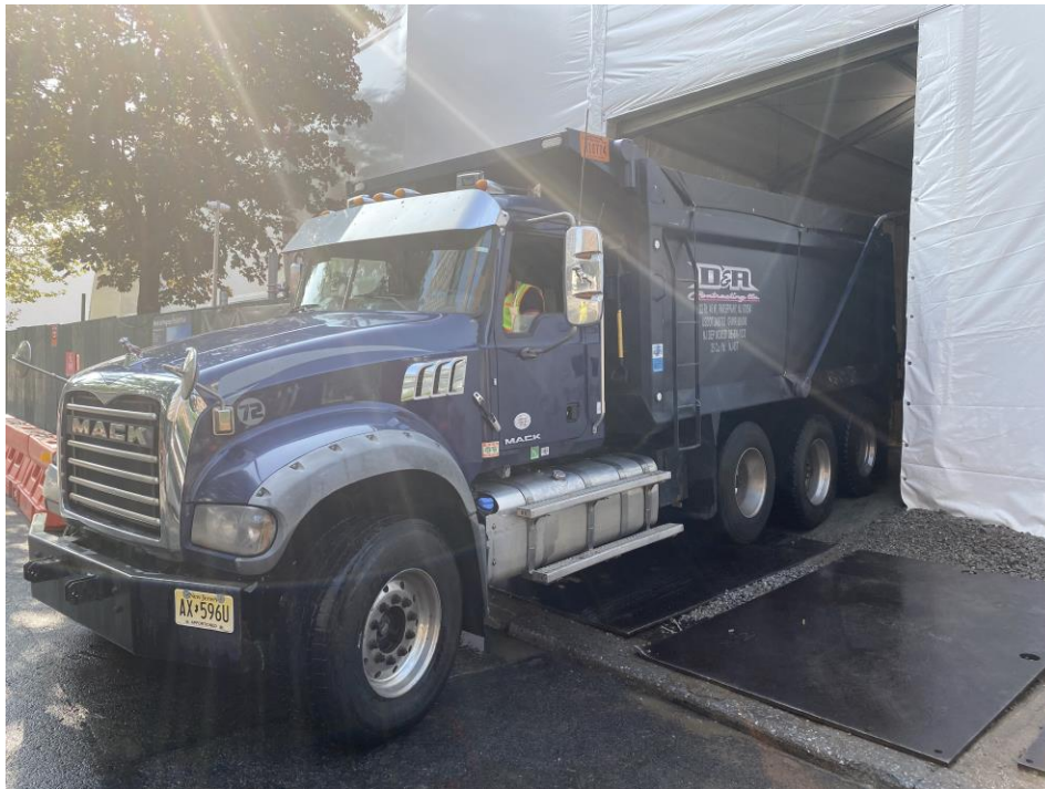
Photo 2: View of truck leaving truck wash station with secured cover, facing southeast.
