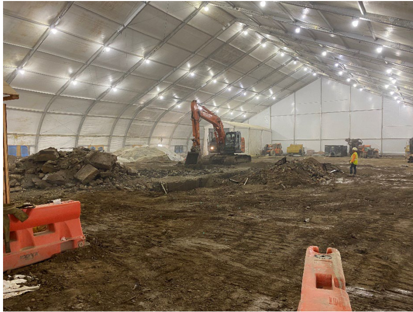
Photo 1: View of slab demolition within enclosure, facing northwest.
