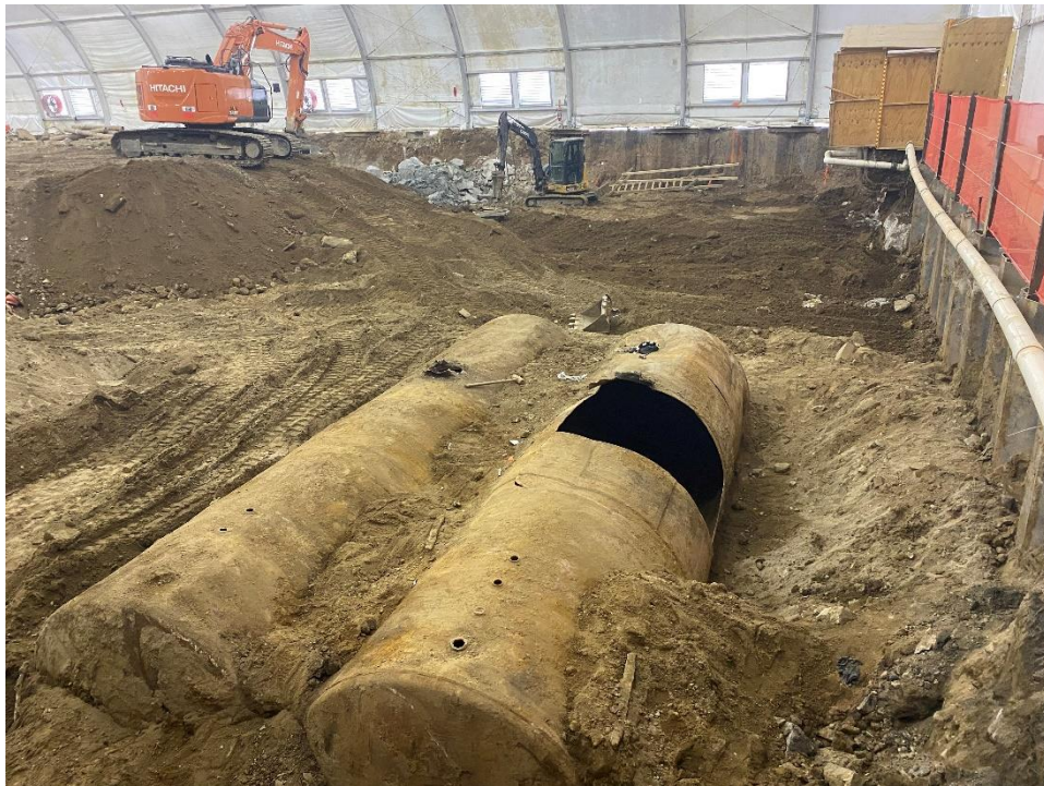
Photo 2: View of TK6 cut open for cleaning and TK7.
