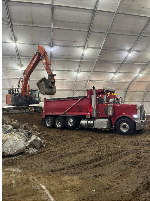
Photo 1: View of loading of soil from 0 to 6 ft bgs within the enclosure.
