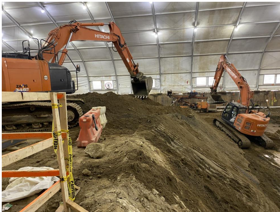
Photo 2: View of excavation within the enclosure.
