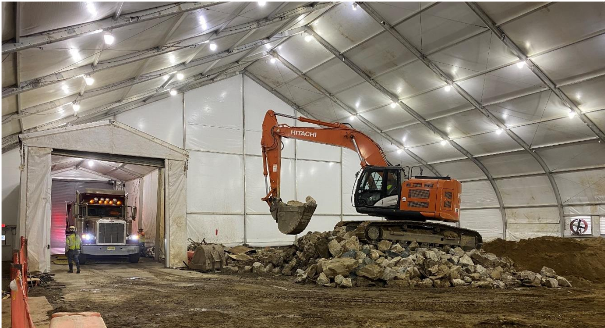
Photo 2: View of concrete truck entering the Site.
