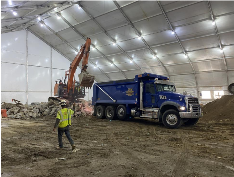
Photo 1: View of C&D debris material loading.
