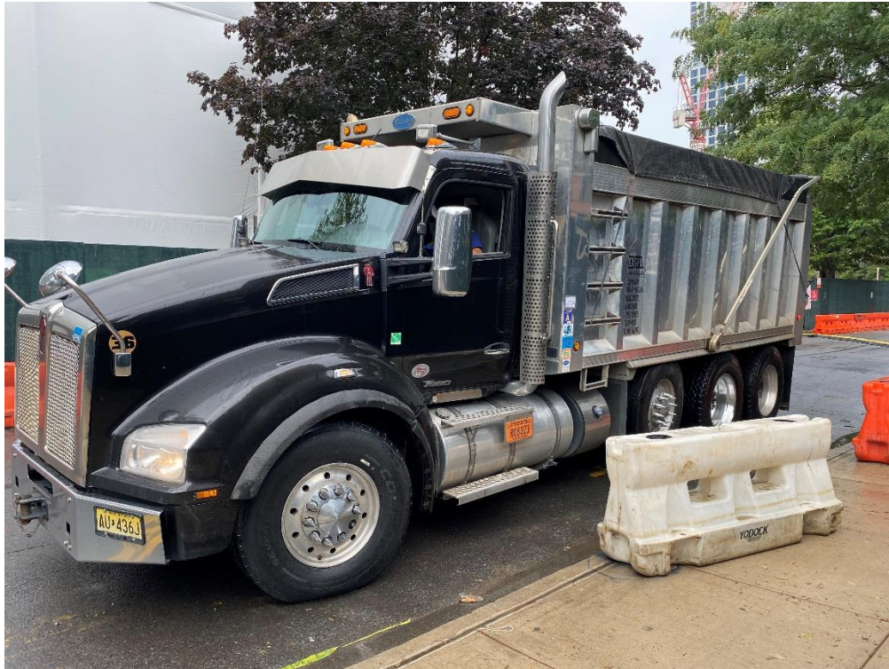
Photo 1: View of secured truck cover and truck exiting Site.
