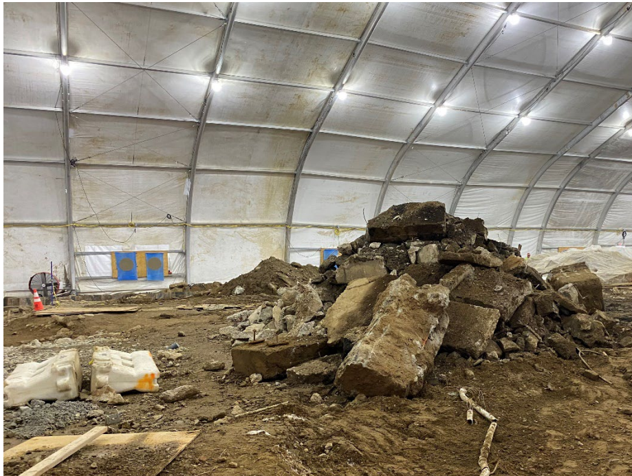
Photo 2: View of slab demolition within enclosure, facing east.
