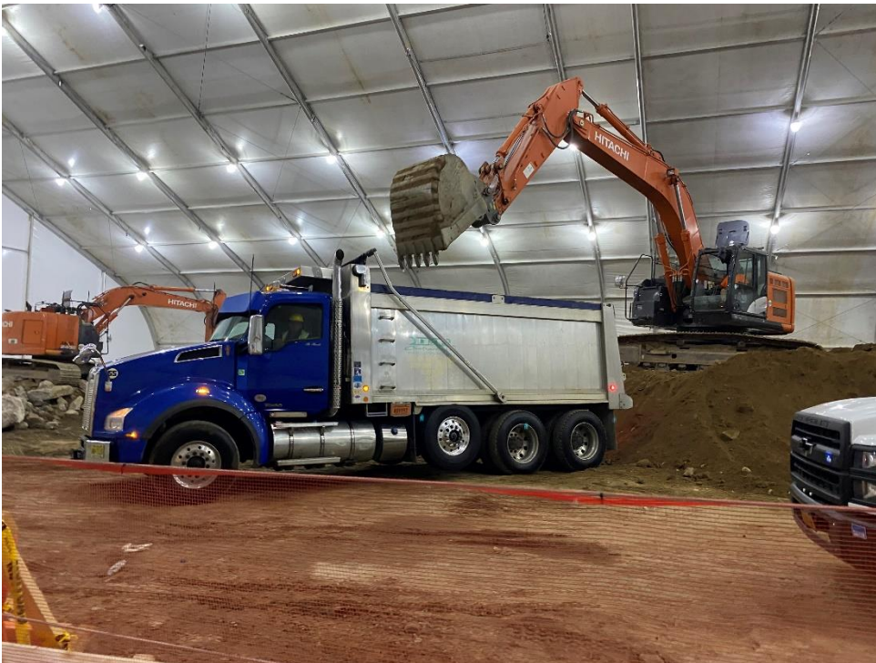
Photo 2: View of soil loading from 0 to 6 ft bgs within the enclosure facing northeast.
