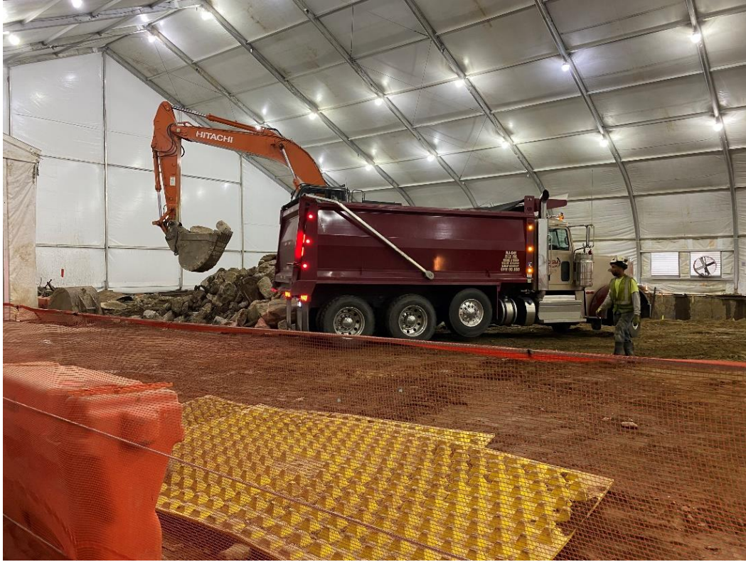
Photo 1: View of C&D debris material loading within the enclosure.
