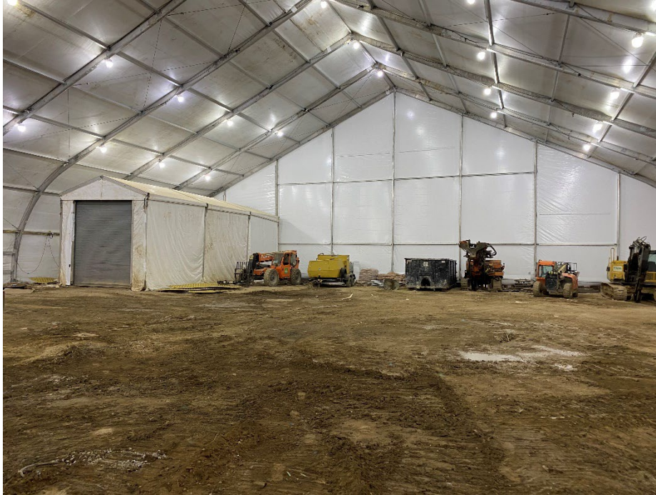
Photo 1: View of site conditions within enclosure, facing north.
