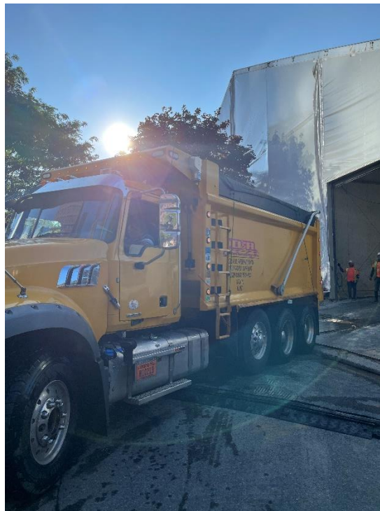
Photo 2: View of covered truck exiting the enclosure.
