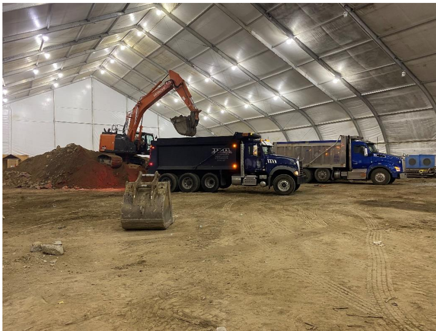
Photo 2: View of truck loading with soil from 0 to 6 ft bgs within the enclosure.
