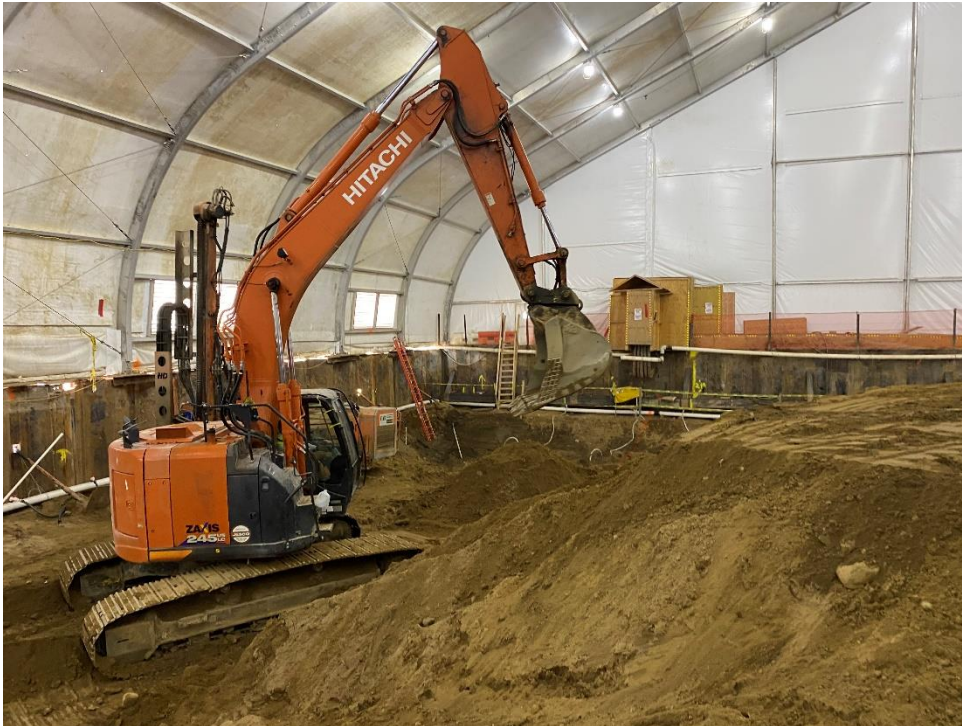
Photo 2: View of soil stockpiling and dewatering system installation facing southeast.
