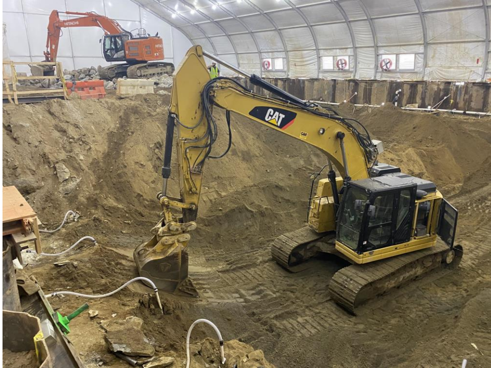
Photo 1: View of excavation within the enclosure.
