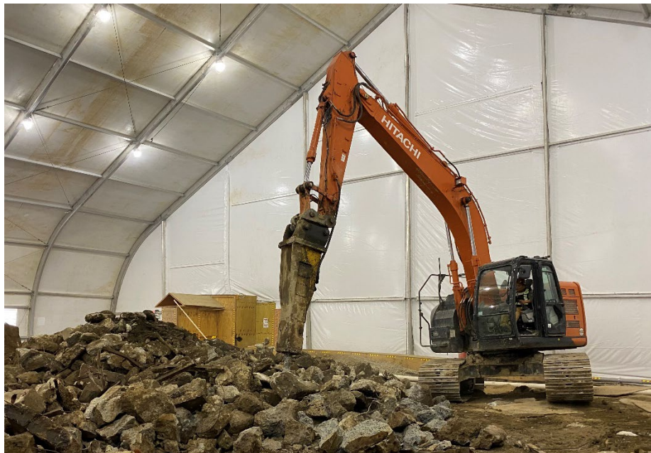
Photo 2: View of slab demolition within enclosure, facing southwest.
