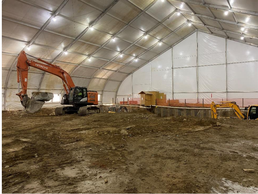
Photo 1: View of site conditions facing south.
