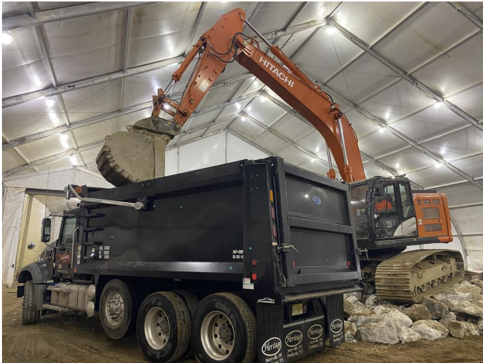
Photo 2: View of C&D debris loading within the enclosure.
