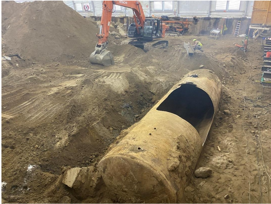
Photo 1: View of TK6 cut open and interior cleaned.
