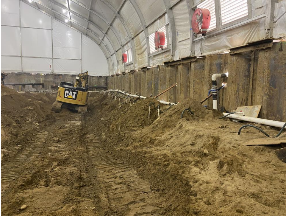
Photo 1: View of excavation and dewatering system within the enclosure.
