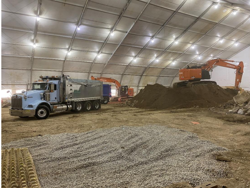
Photo 1: View of truck loading with soil from 0 to 6 ft bgs.
