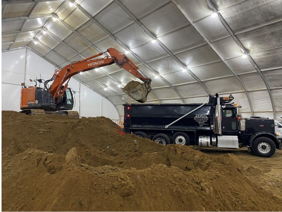
Photo 1: View of soil loading with stockpiled soil from 0 to 6 ft bgs.
