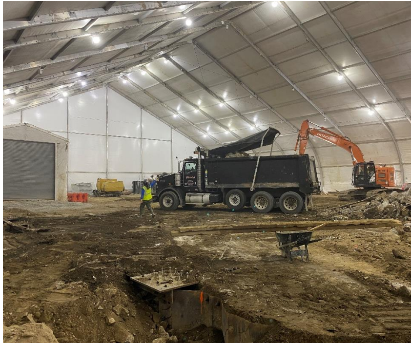
Photo 1: View of C&D debris material loading within enclosure, facing northeast.
