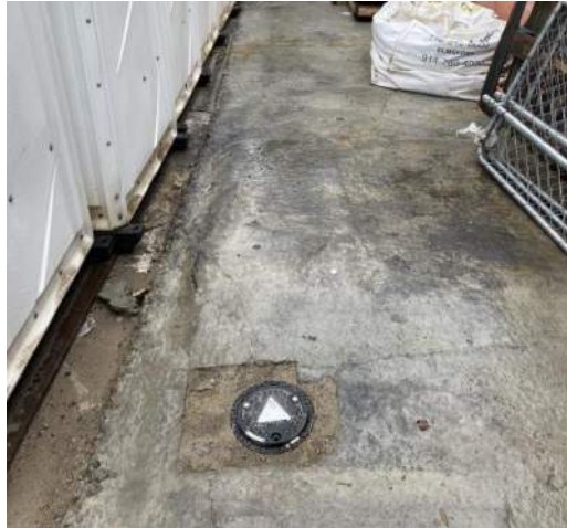
Photo 1: View of recovery well RW-25 located on the Franklin Street sidewalk within the construction fencing.
