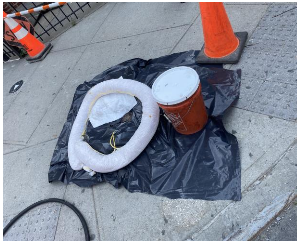
Photo 9: View of spill containment setup at MW-26 on the southeast corner of Dupont and Franklin Street.
