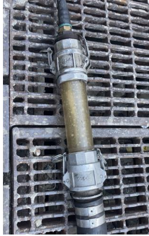
Photo 7: View of groundwater extraction passing through transparent pipe section of vac truck flexible hose.
