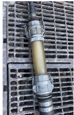
Photo 6: View of groundwater extraction passing through transparent pipe section of vac truck flexible hose.
