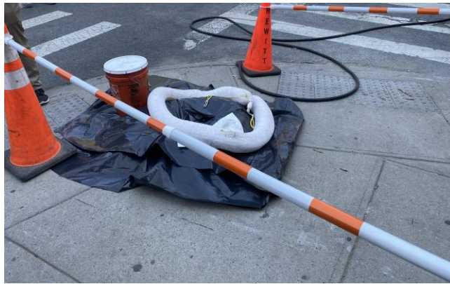
Photo 8: View of spill containment setup and pedestrian delineation at MW-26 on the southeast corner of Dupont and Franklin Street.
