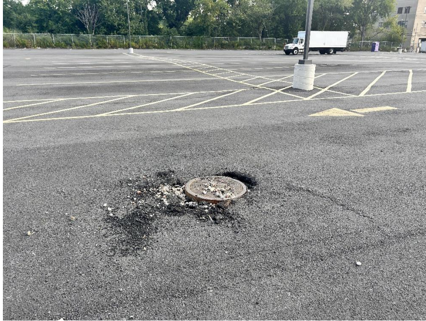
Photo 7: Spalling asphalt around manhole cover in the central part of the site (facing northeast).
