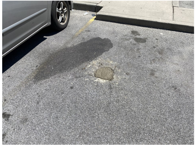
Photo of MW-2, decommissioned and concreted to the ground surface.
