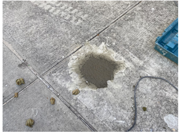
Photo of MW-8, decommissioned and concreted to the ground surface.
