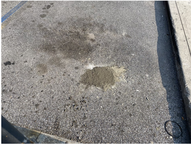
Photo of MW-7, decommissioned and concreted to the ground surface.
