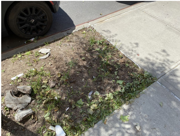
Photo of MW-9, decommissioned and backfilled to the ground surface.
