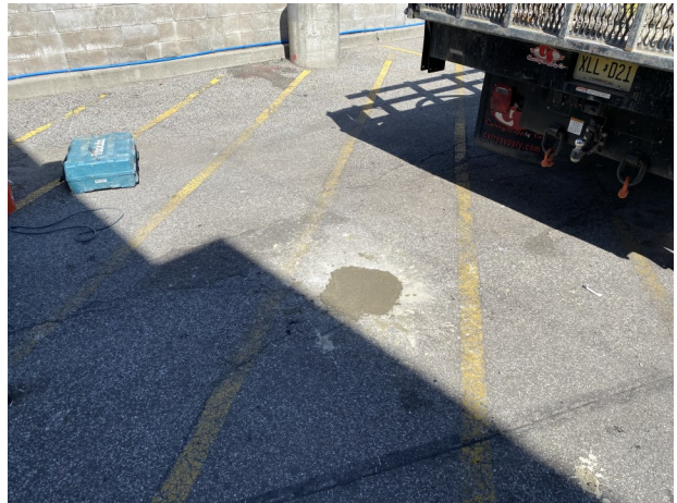
Photo of MW-4, decommissioned and concreted to the ground surface.
