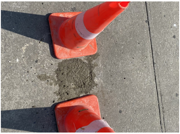
Photo of MW-6, decommissioned and concreted to ground surface.
