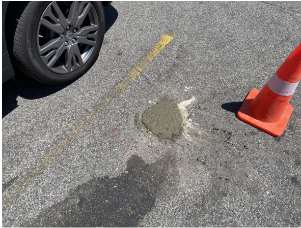
Photo of MW-1, decommissioned and concreted to the ground surface.
