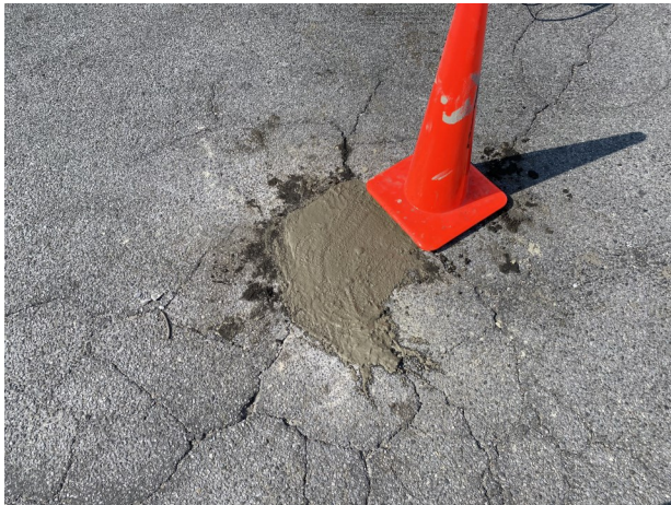
Photo of MW-3, decommissioned and concreted to ground surface.
