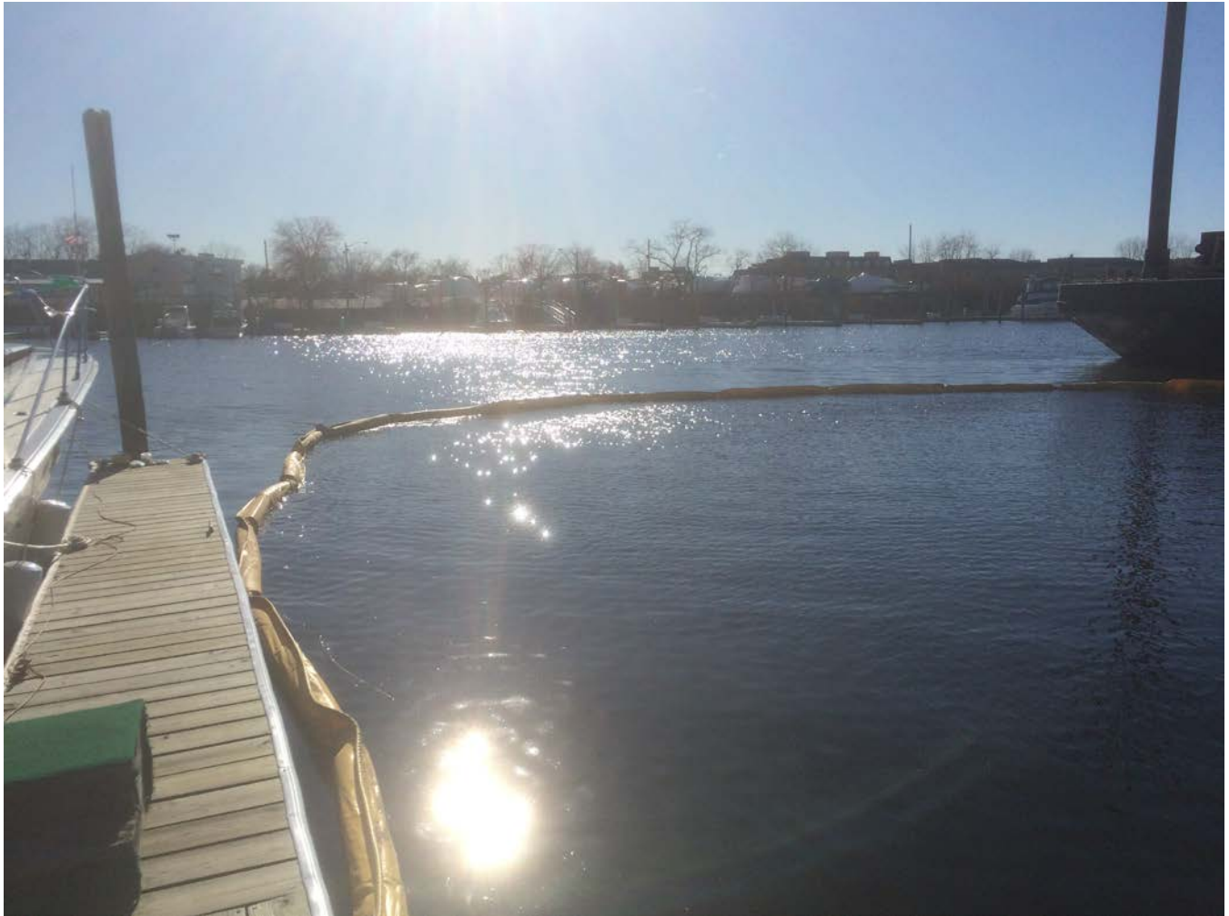
Photo 2: Turbidity Curtain and Barge Facing SW
