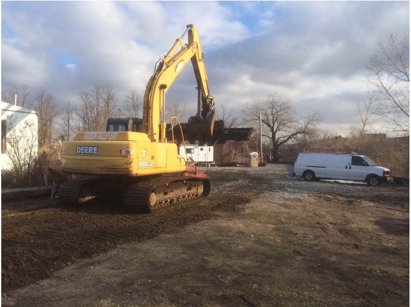
Photo 2: Excavator Carrying Floating Dock Material to Drying Pad Facing NE
