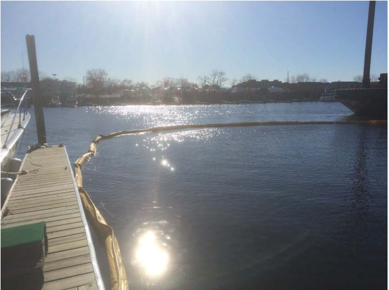
Photo 2: Turbidity Curtain and Barge Facing SW
