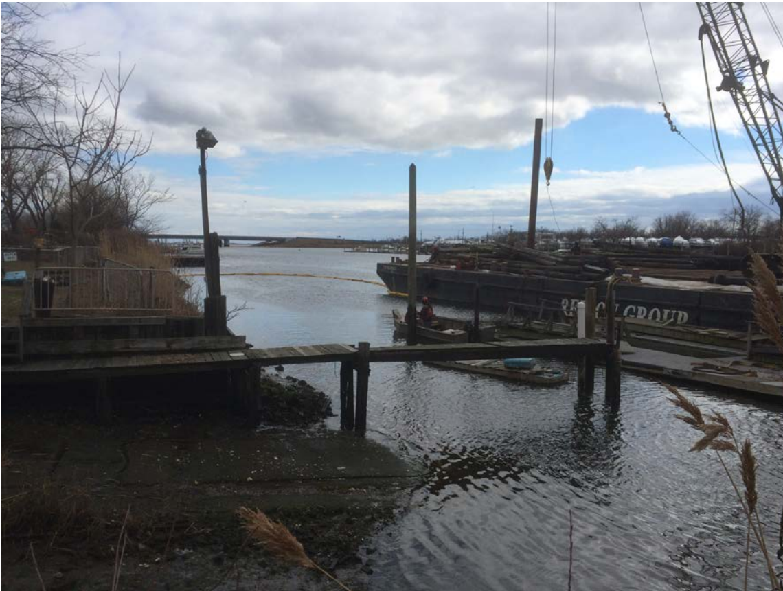
Photo 1: Barge and Turbidity Curtain S
