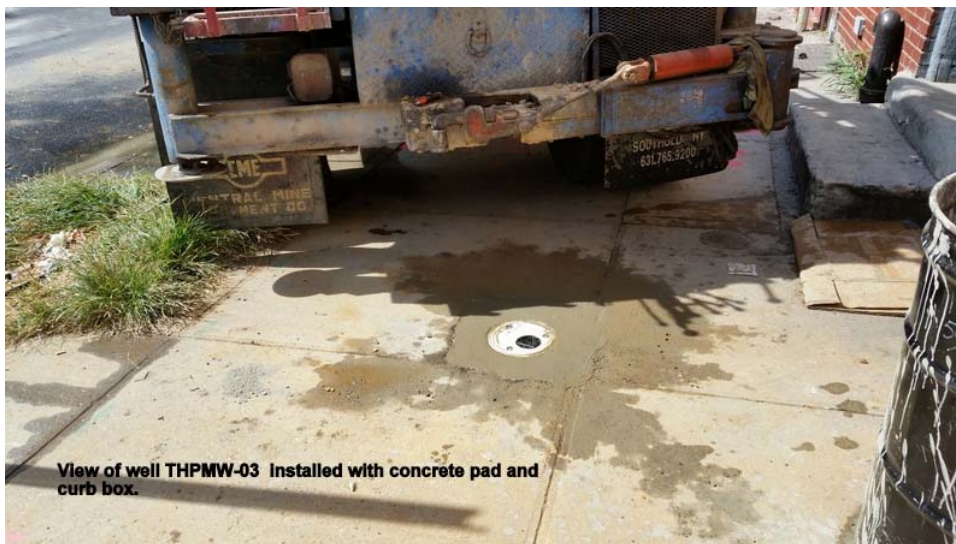
View of well THPMW-01 installed with concrete pad and curb box.
