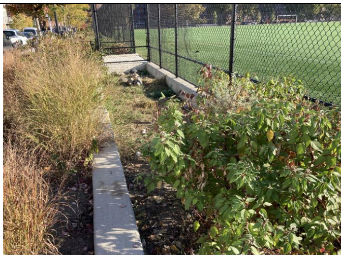
Photo 3: Additional mulch and grasses needed at Bioswale Area along Hicks Street.
