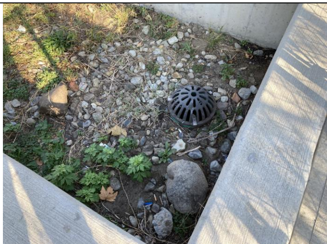
Photo 11: Additional mulch and grasses needed at Bioswale Area along Bay Street.
