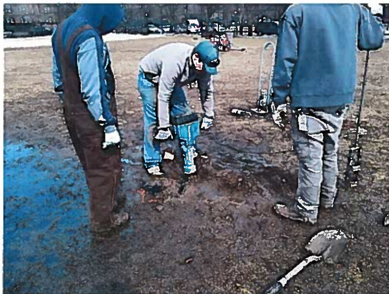
Using jack hammer to dislodge debris at 18 to 24 inch depth at SS008
