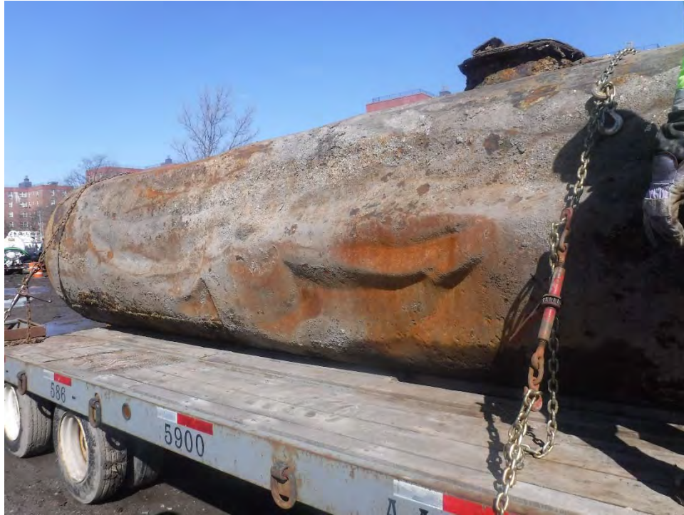
Photograph No. 7: After cleaning of the UST and inspection, the UST was loaded onto a flatbed trailer and transported to Benson Scrap Metal ((718)-722-7754) at 543 Smith Street, Brooklyn, New York for recycling.
