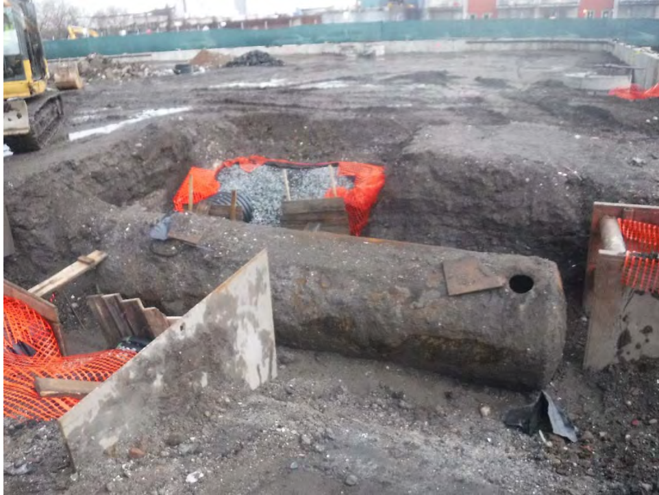
Photograph No. 1: View of the UST exposed prior to its removal from 98 Lorraine Street, Brooklyn, New York. The property is an empty lot formerly used as a smelting facility. The UST closure activities were conducted by AARCO, with oversight by AECOM, and the New York City Parks Department.
