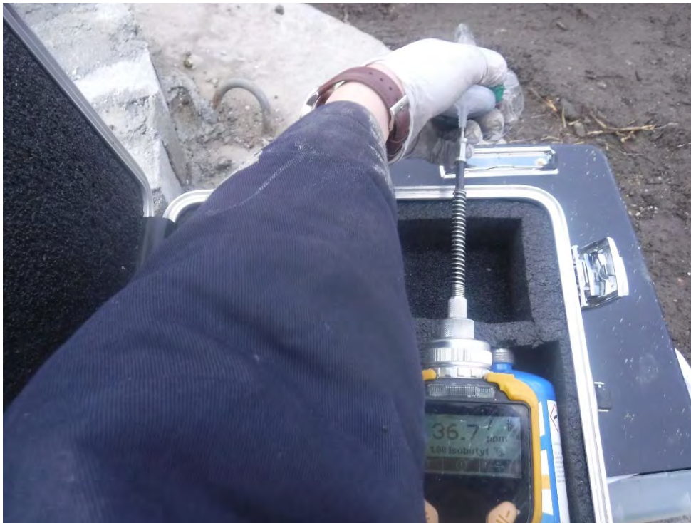
Photograph No. 6: After the UST was removed from the ground, Preferred's Field Geologist screened soils along the bottom and sidewalls of the excavation for visual or olfactory evidence of petroleum impacts, as well as for the presence of VOCs utilizing a PID. Petroleum odors and elevated PID responses up to 96.1 Parts Per Million (PPM) Response Units (RUs) were noted in soils along the bottom of the excavation.
