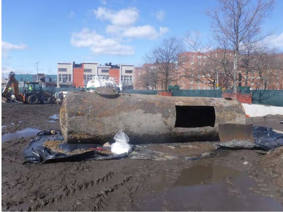
Photograph No. 3: After extracting the UST from the ground, same was temporarily staged adjacent to the excavation on top of plastic sheeting. A hole was cut in the side of the UST to allow for cleaning of the interior and inspection.
