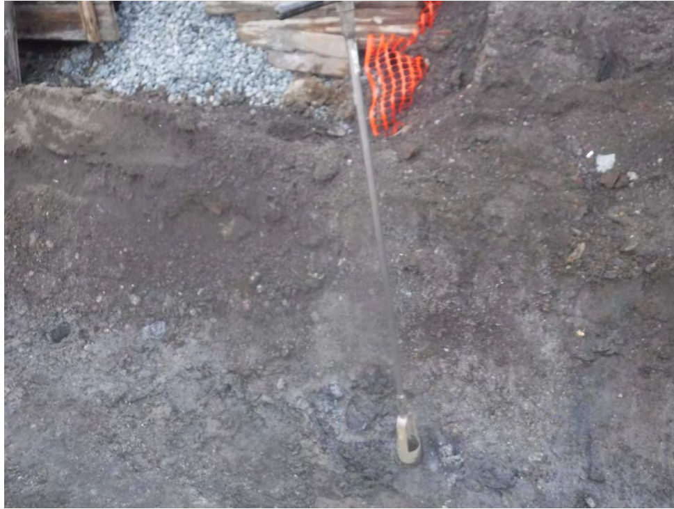
Photograph No. 5: A stainless steel hand auger was utilized to collect six (6) bottom and sidewall samples from the former tank location. These samples were sent for laboratory analysis.
