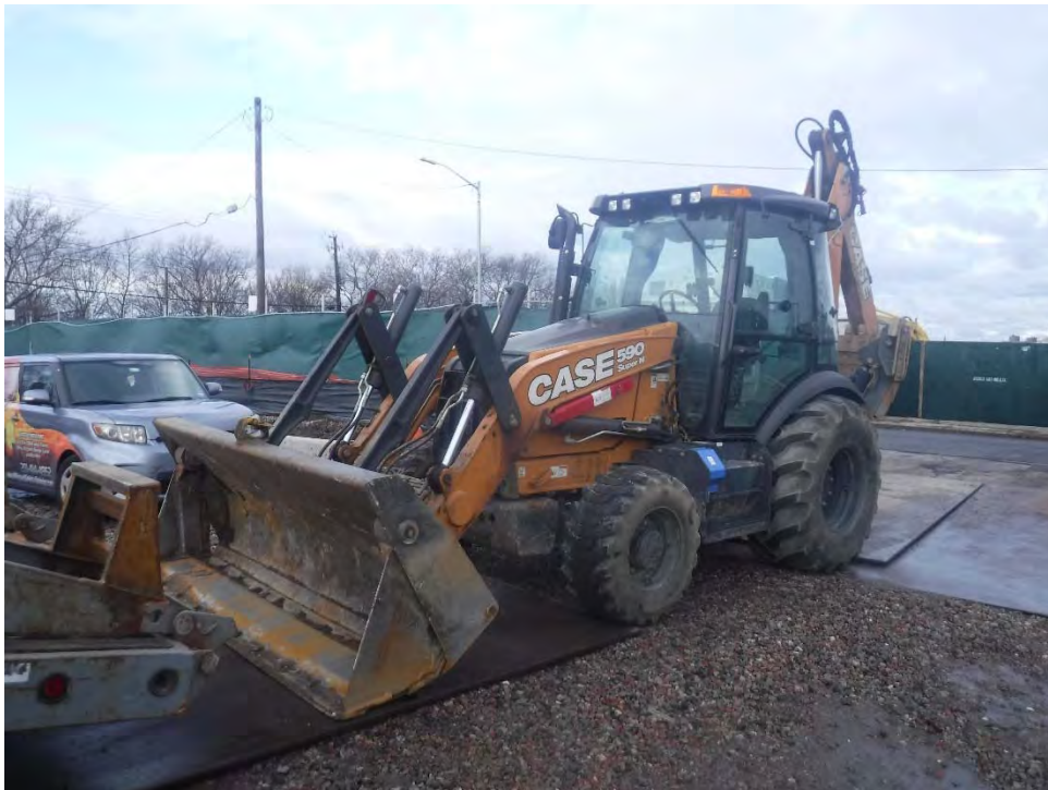
Photograph No. 2: A Case 590 Super N excavator was utilized to remove the UST.
