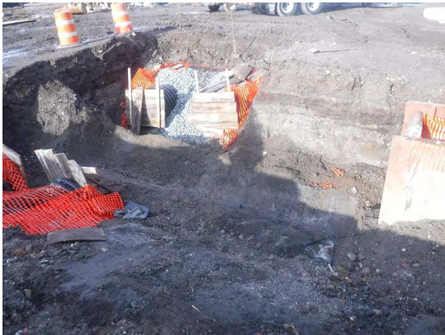
Photograph No. 8: View of the Excavation area after the tank removal and soil sampling.
