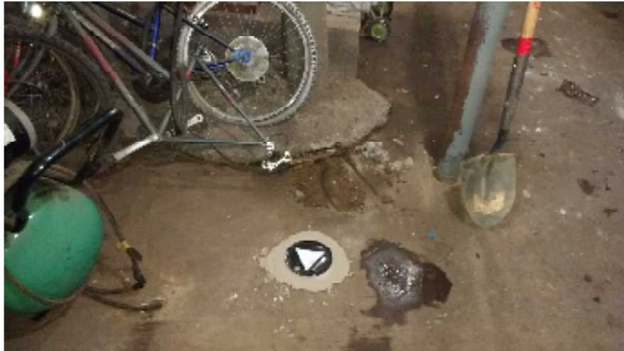
Well MW-1 Completion in Flush-mount Box
