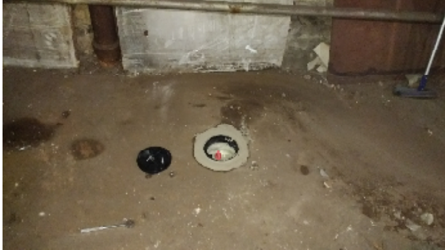
Finished Well MW-2 along West Wall
