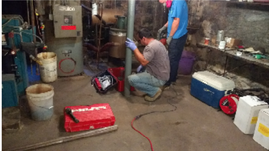
Drilling SV-1 Near Boilers
