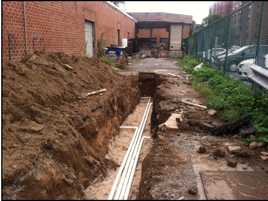
Photo 3: The piping at the lower left of the photo runs in from the east end of the trench, then turns south toward the parking lot, and then upwards, above ground, for connection to the remediation compound.
