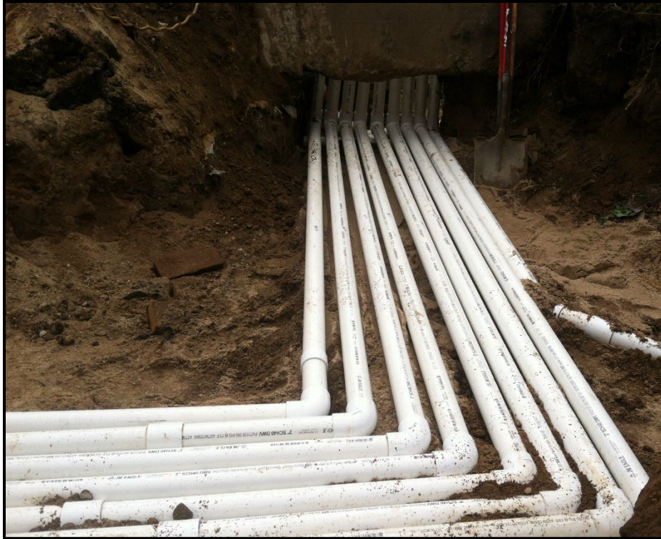
Photo 2: View of east end of the trench and piping and connections to wells AS-3 and AS-4 to the right, and wells SVE-6 and SVE-7 to the left. The trench was underlain with four inches of clean sand prior to installing the pipes.
