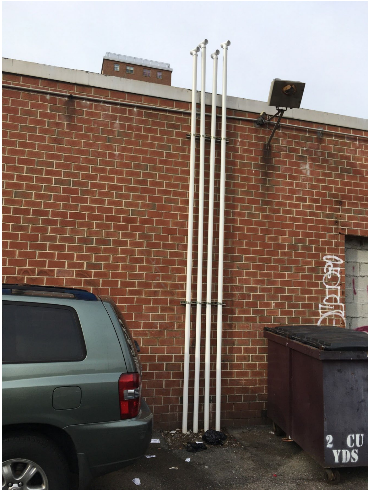
Photograph of one of the two clusters of exhaust pipes along the rear wall of the building.
