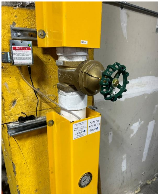
Labels placed on steel guards at approximately 4-feet high
