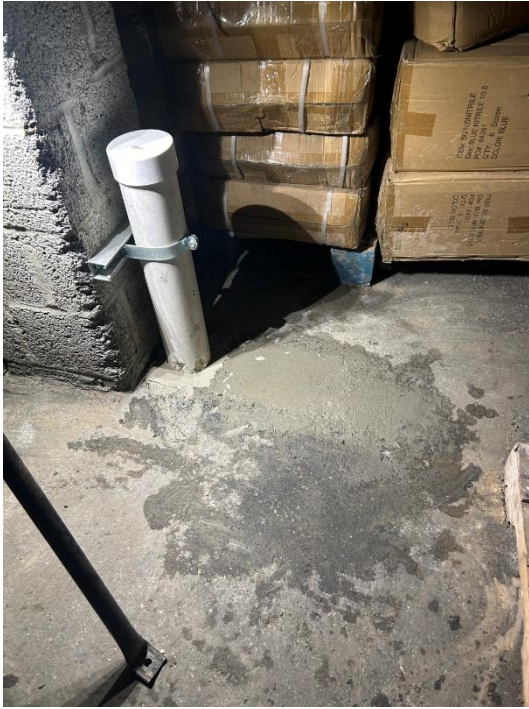
SP-3 installed along existing column with pipe pathway open between shelving
