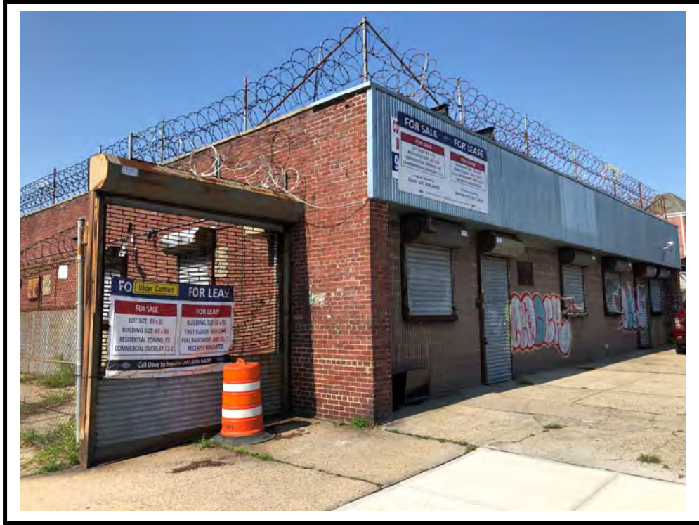
PHOTO LOCATION: Depicts facing west to the front of the subject property.
