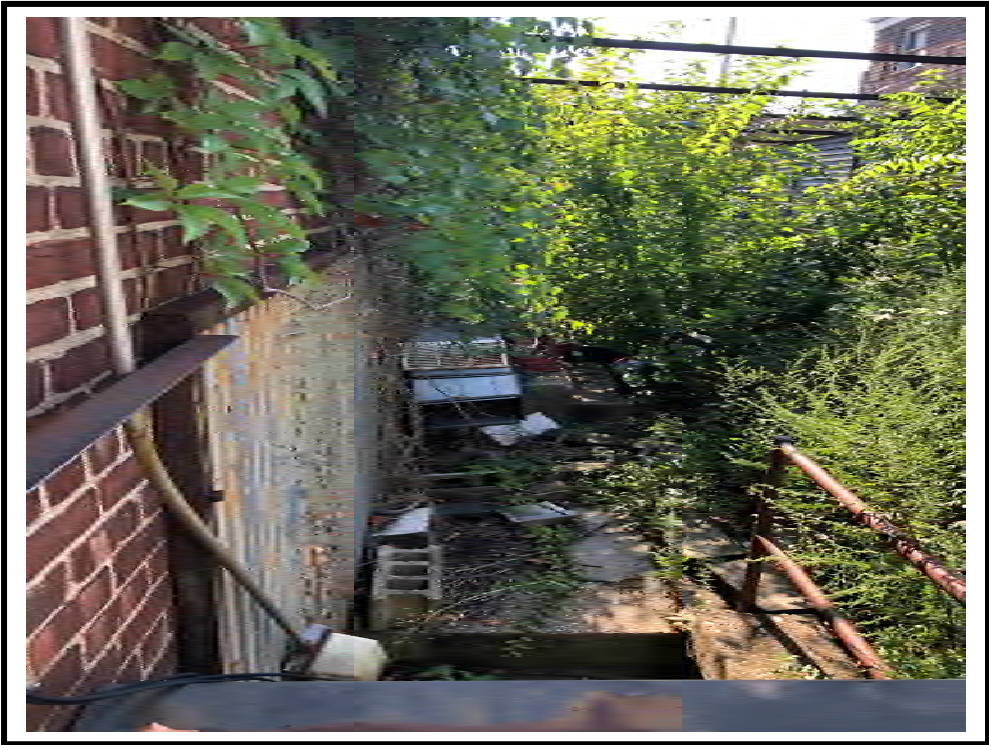
PHOTO LOCATION: Depicts overgrown foliage with various debris and waste in the rear of the subject property.
