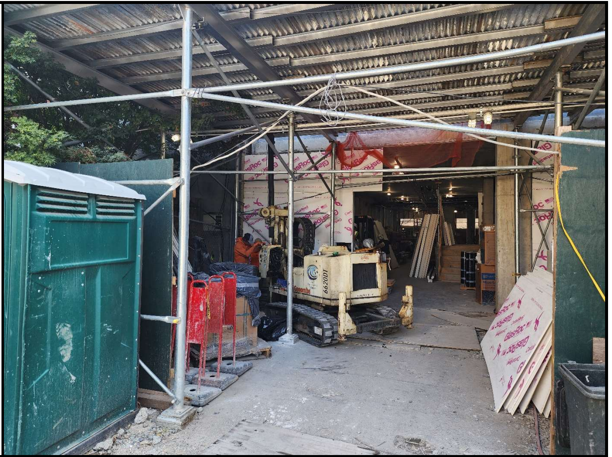
Photo 3 – View of drilling at GW1 location
