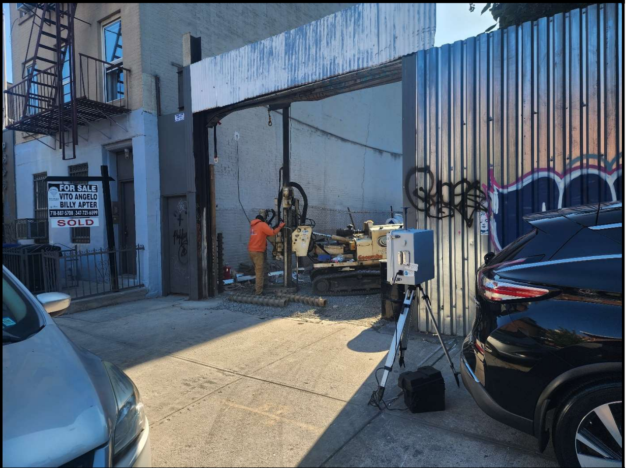
Photo 1 – View of drilling at GW2 location
