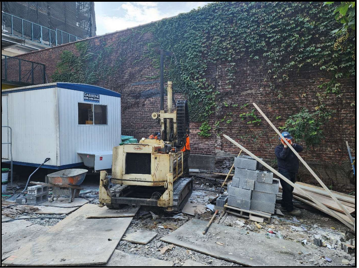
Photo 1 – View of drilling at SB5 location
