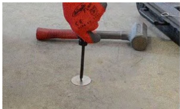
Figure 5. Tightening the Secured Cover
