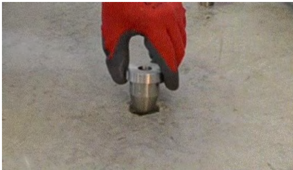
Figure 3. Testing Depth with the Drilling Guide
