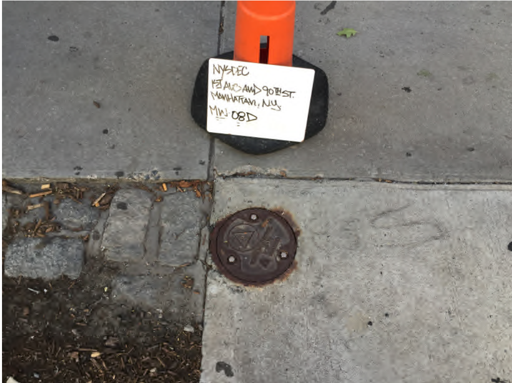
Photograph 7: Condition of MW-8D
