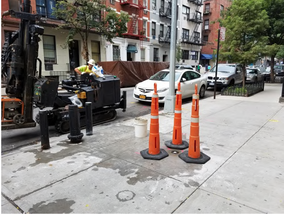
Photograph 3: View of VP126 completed.
