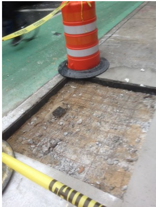
Photograph 10: Sidewalk replacement of SG-016 along 2 nd Avenue.
