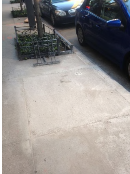
Photograph 13: Sidewalk replacement with larger manhole (SG-079)
