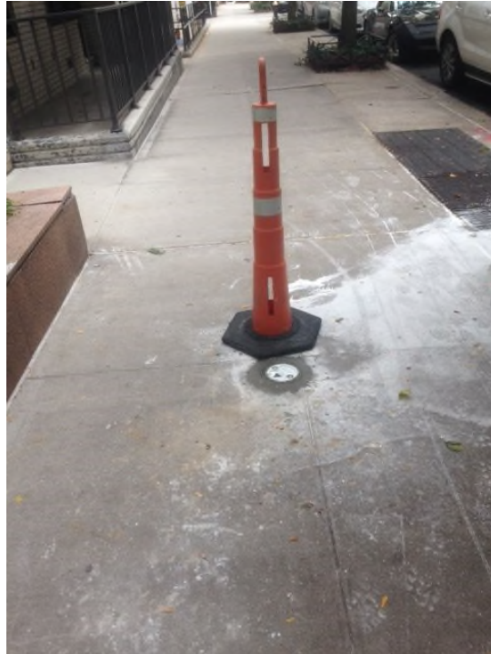
Photograph 9: Installation of larger manhole at SG-076 along 1 st Avenue.
