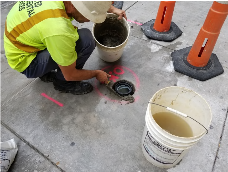
Photograph 2: Installation of manhole at VP126.
