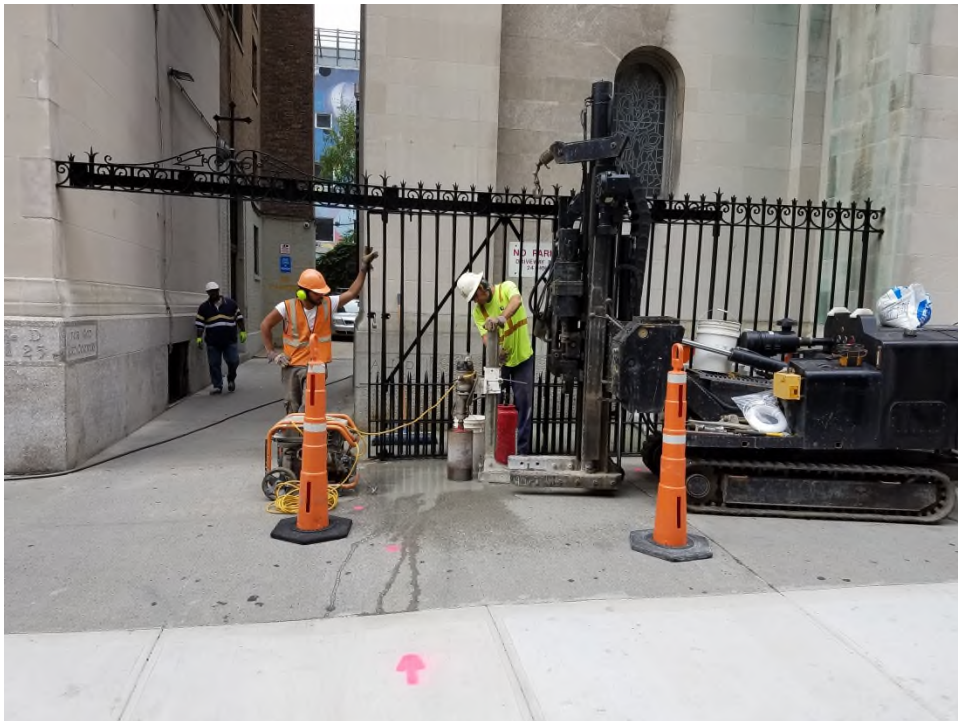
Photograph 4: Coring of concrete at VP129 along East 87 th Street.
