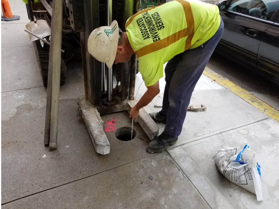
Photograph 7: Installation of the soil vapor implant and tubing at VP130.
