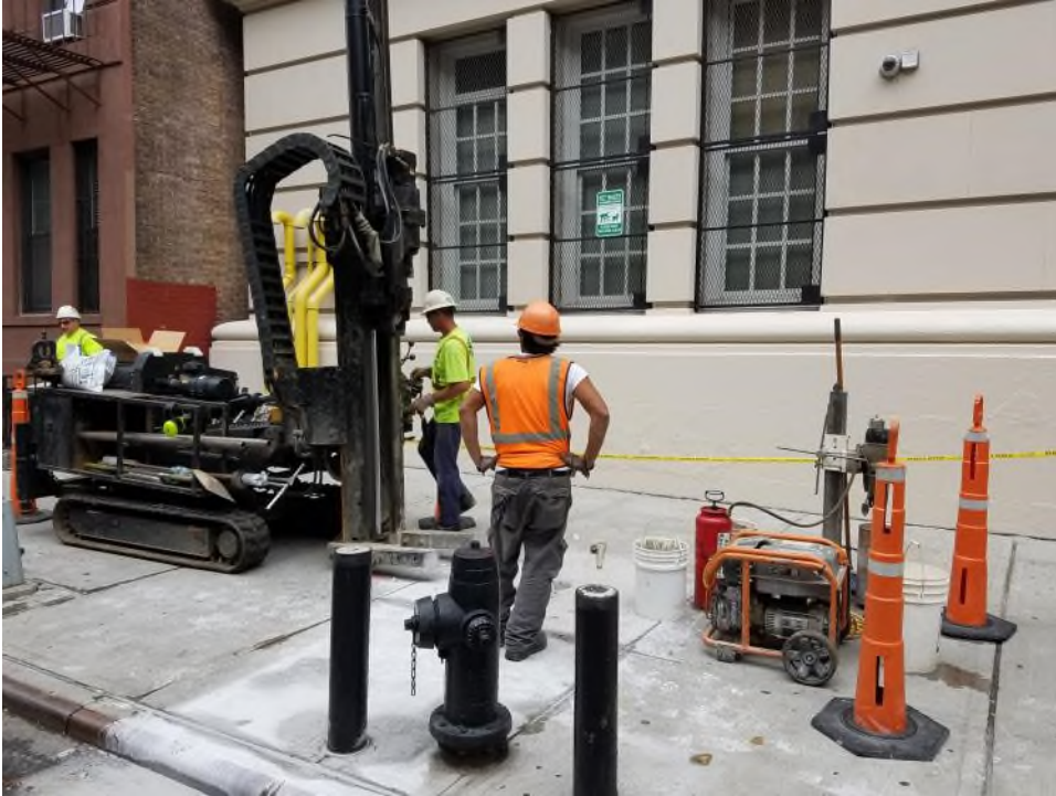
Photograph 1: Installation of soil vapor point VP126 along East 88 th Street.
