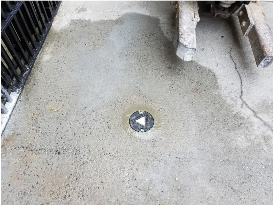
Photograph 6: View of VP129 completed.
