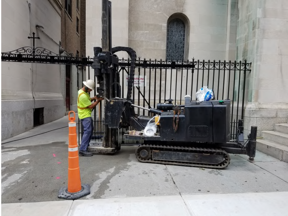
Photograph 5: Installation of VP129 via Geoprobe.
