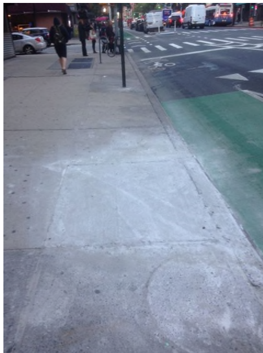
Photograph 14: Sidewalk replacement (VP-128)
