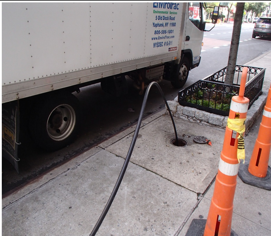
Photograph 5: “Tremie” pipe used to decommission monitoring wells.
