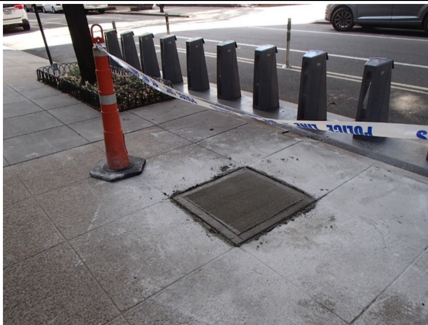
Photograph 13: Finished sidewalk flag replacement.
