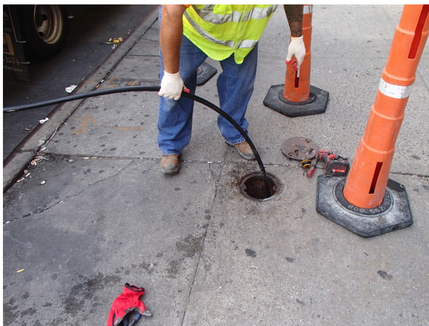
Photograph 4: Decommissioning of groundwater monitoring well.
