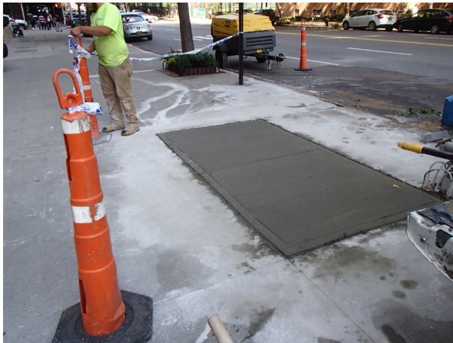
Photograph 12: Finished sidewalk flag replacements.
