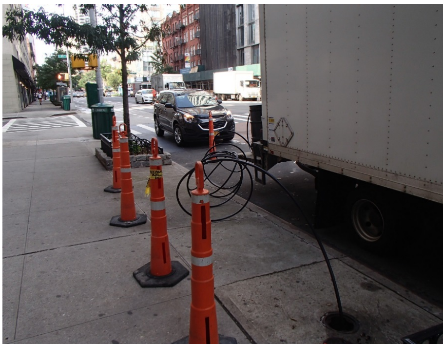
Photograph 6: Abandonment of groundwater monitoring well.
