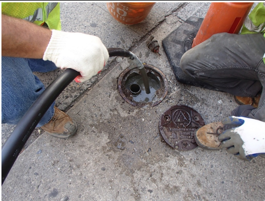
Photograph 7: View of groundwater monitoring well abandonment in place.
