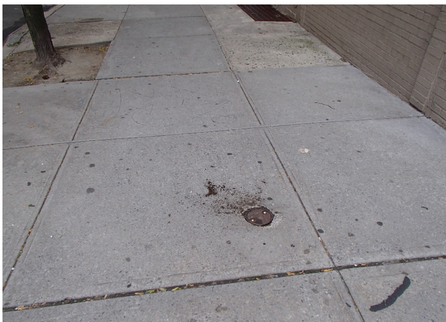
Photograph 8: Soil gas point abandoned in place with cover.
