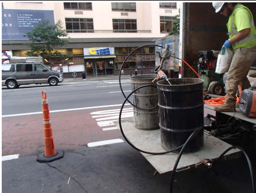
Photograph 3: Grout mixing for groundwater monitoring well abandonments.
