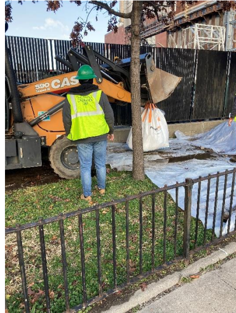
Photo 6 – View of soil in powerpaks being transported.
