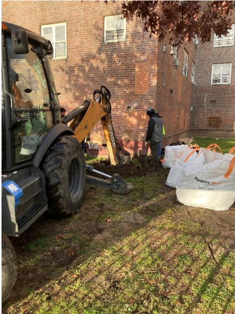
Photo 5 – View of excavation near building.
