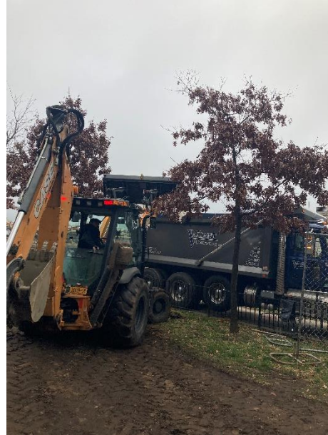
Photo 10 – View of excavator loading soil for offsite transport and disposal.
