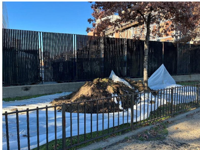
Photo 3 – View of temporary soil pile on poly sheeting.
