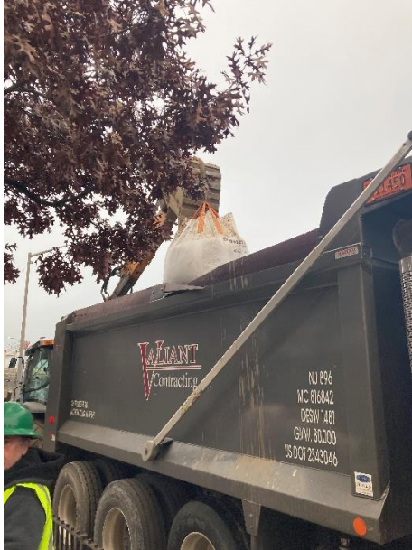
Photo 9 – View of powerpaks being loaded for offsite transport and disposal.
