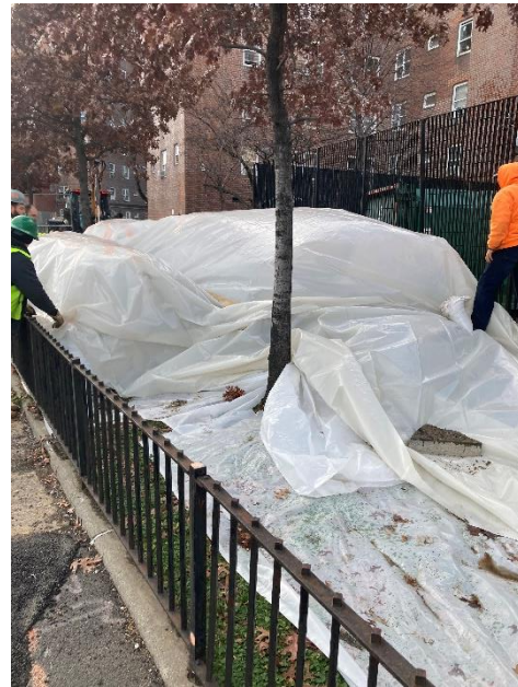
Photo 8 – View of soil stockpile covered in poly.
