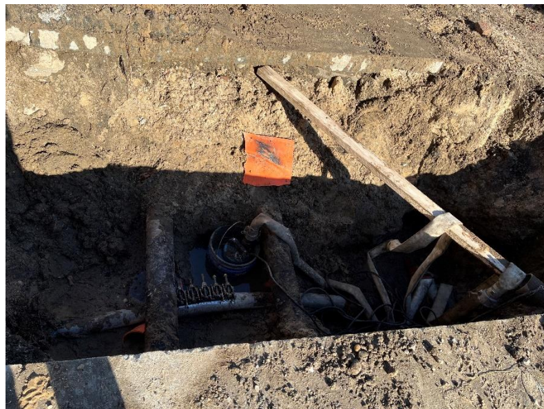
Photo 4 – View of excavation within sidewalk.
