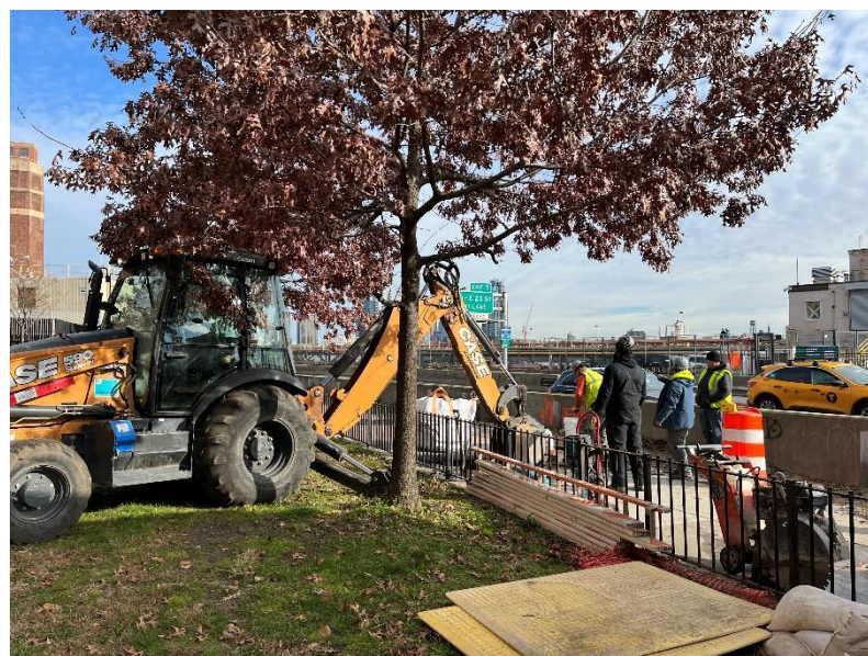
Photo 1 – View of beginning of excavation.
