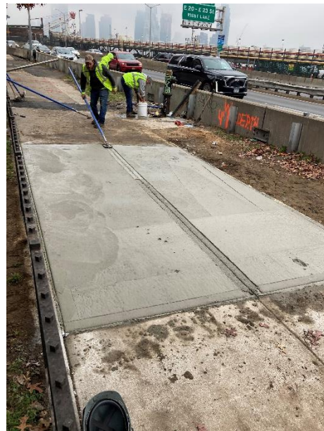
Photo 12 – View of poured concrete sidewalk.
