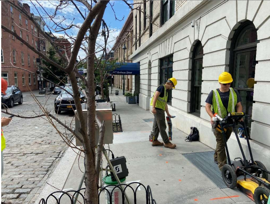
Photo 1: Nova performing utility locating survey on western sidewalk of Beekman Street.
