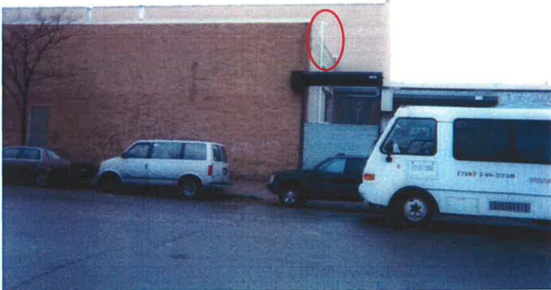
Photograph 7: View of effluent discharge for treated air from SVE system.
