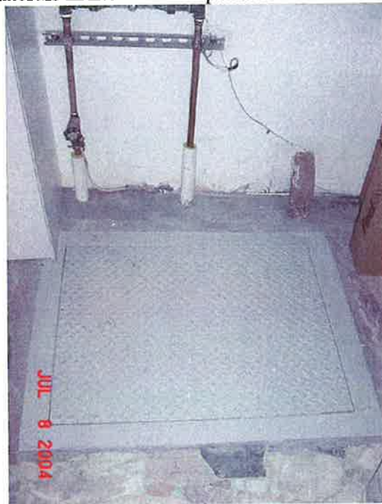
Photograph 4: View of sealed potential vapor migration pathway in office area.
