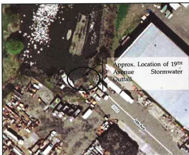
Photograph 1: Stormwater Discharge Sample Location
