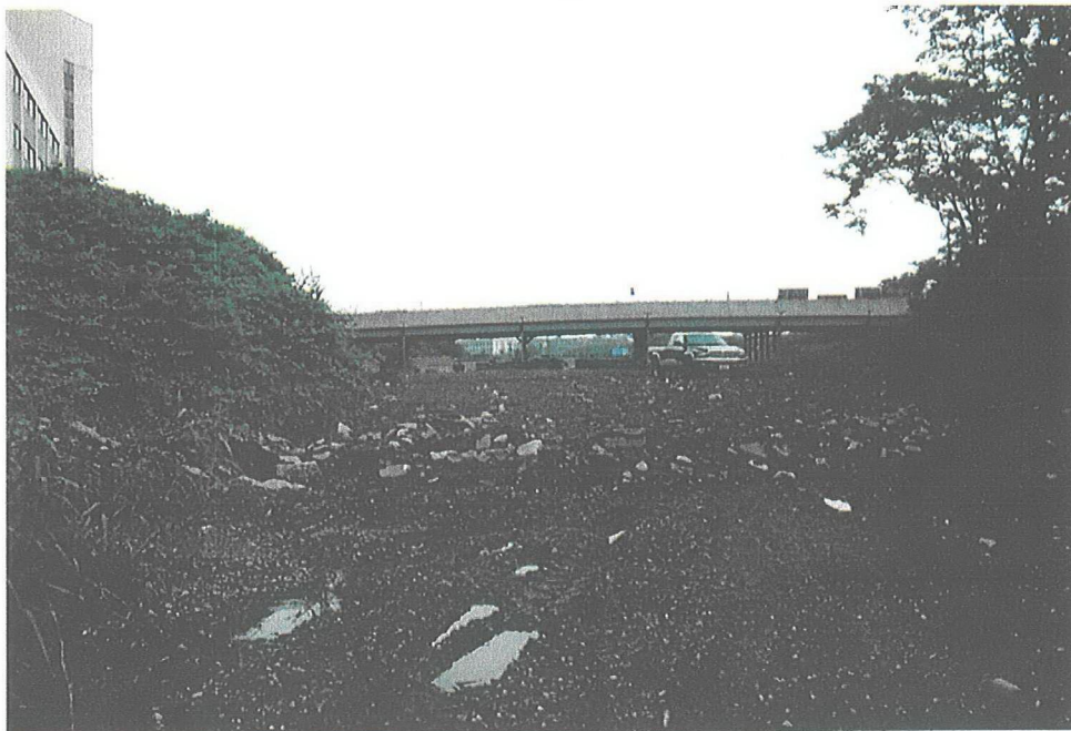
PHOTO 3: East towards 21 st Ave. overpass.
