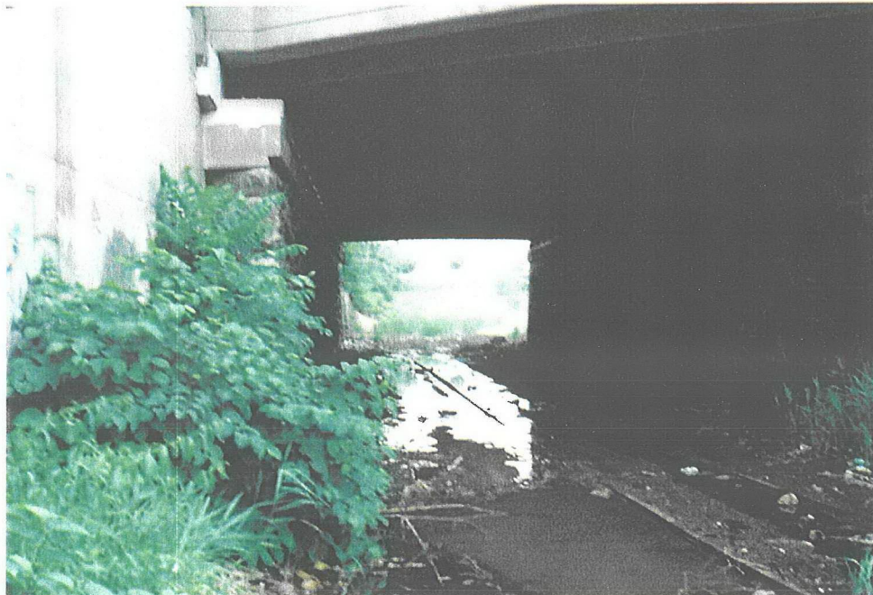
PHOTO 2: Jackson Ave. overpass. Low point of proposed fill area.
