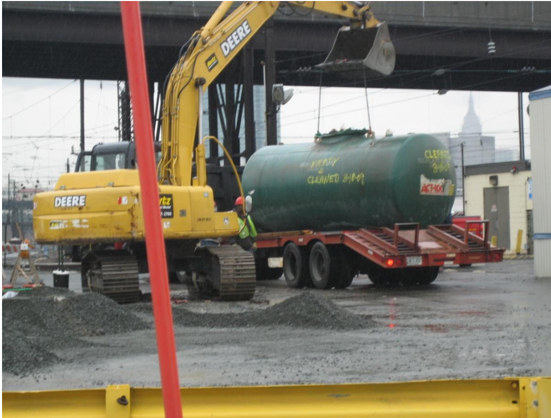
Photograph 15: Tank being loaded for transportation offsite
