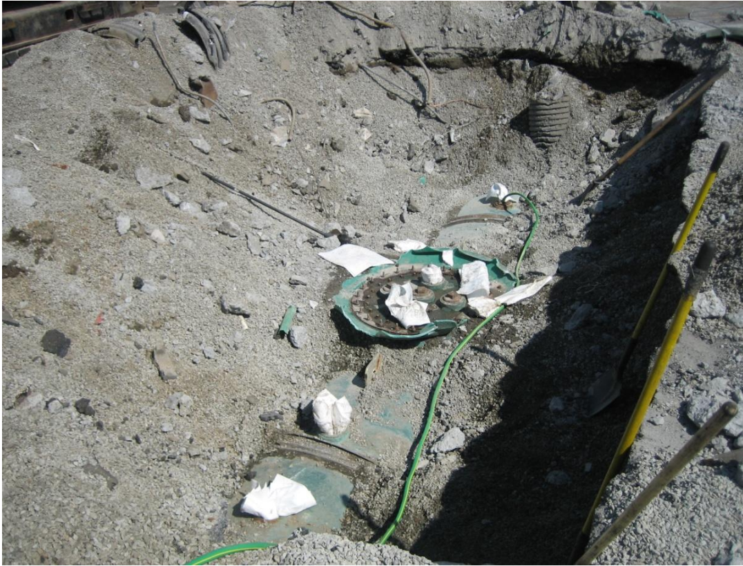
Photograph 5: Preparing to clean the inside of the tank
