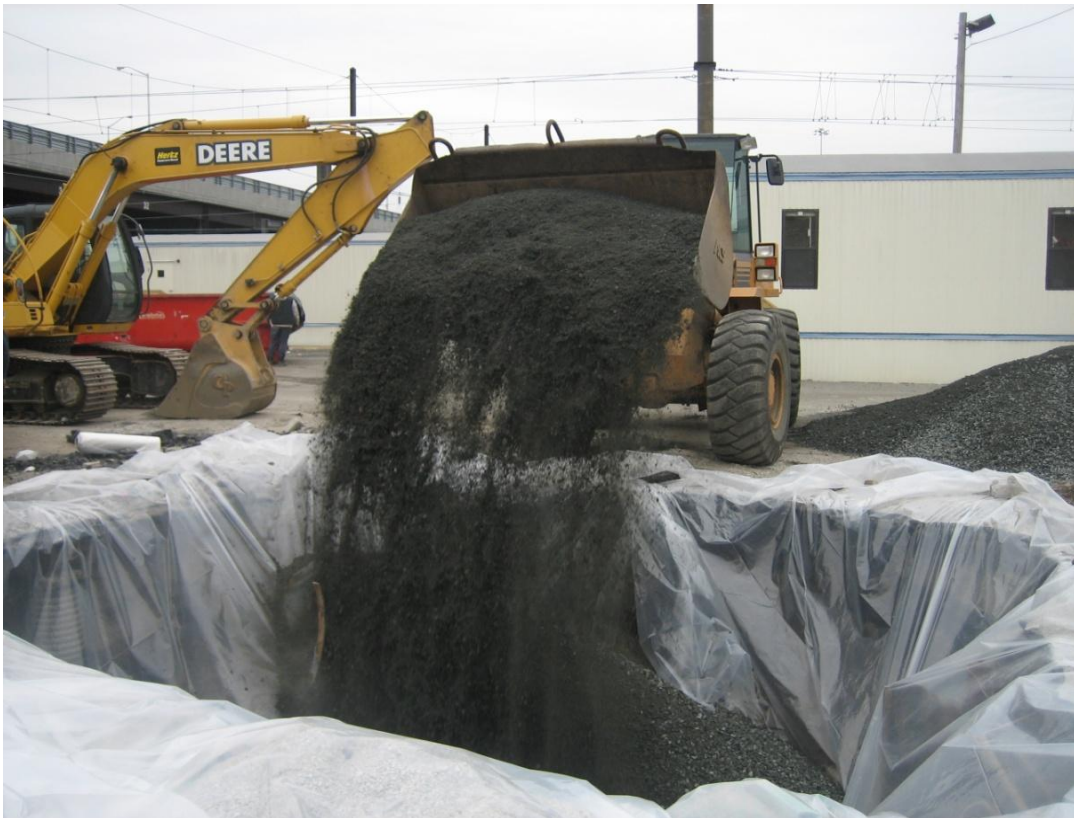
Photograph 14: Backfilling excavation
