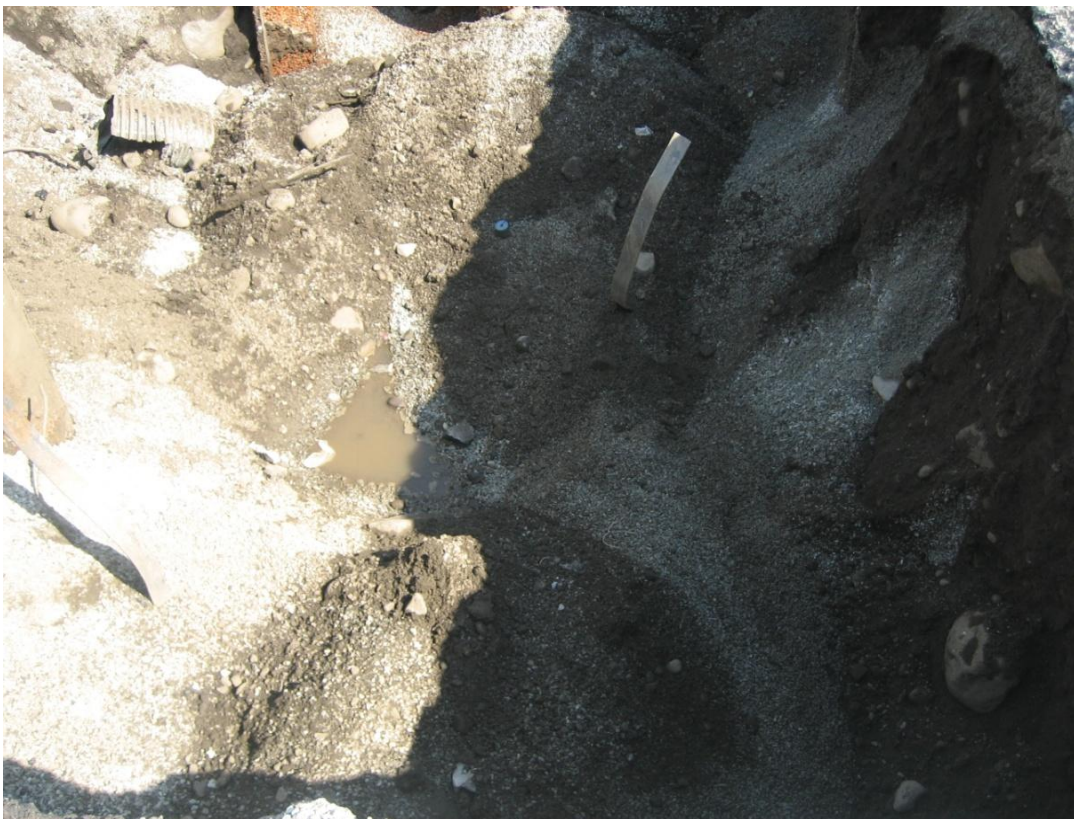
Photograph 12: Groundwater collecting in bottom of excavation
