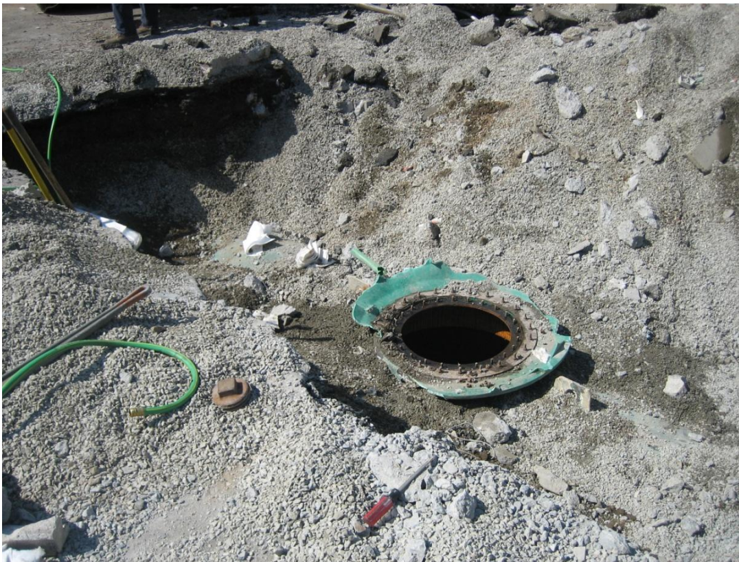
Photograph 6: Open manway used to access tank for cleaning
