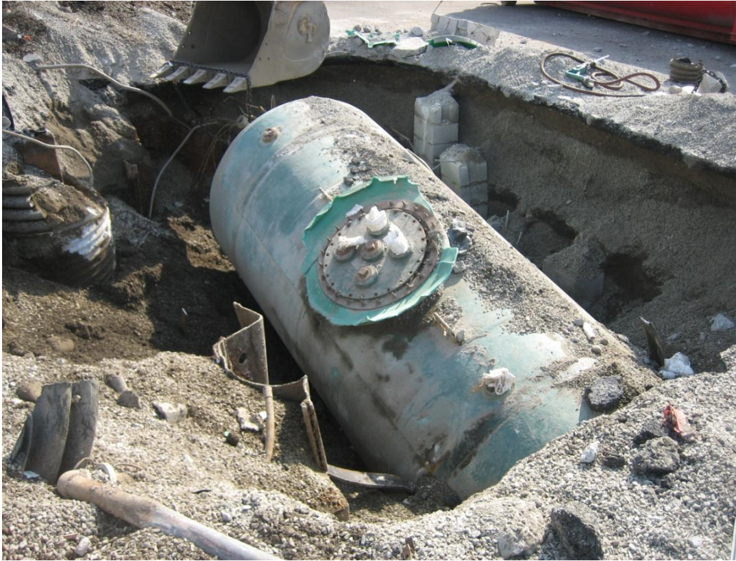
Photograph 7: Tank being removed
