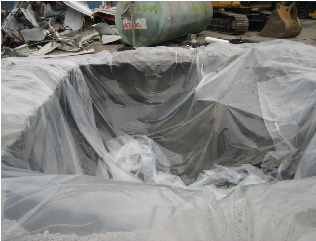
Photograph 13: Excavation lined with poly sheeting prior to backfill
